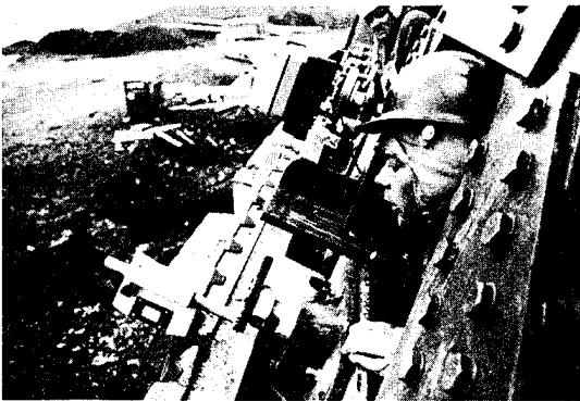
Figure 8. Adjustment of Jack Screws
