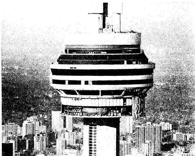
FIG. NO. 8 CN TOWER RADOME INSTALLATION
