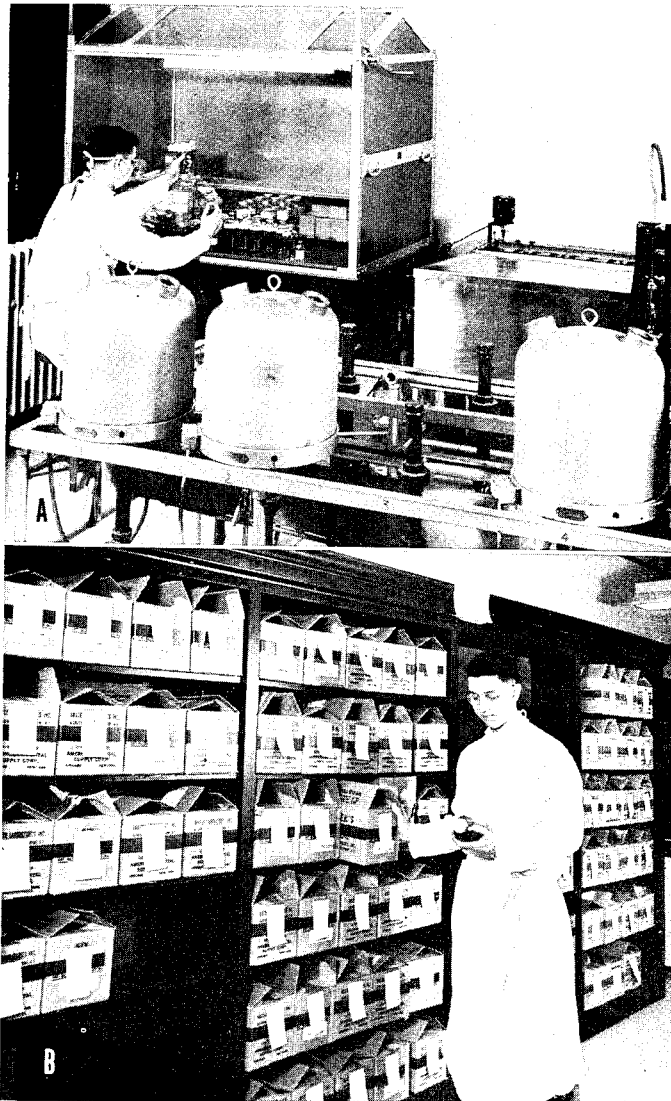
FIGURE 10.—Preparation of liquid plasma, Blood Research Division, Division of Surgical Physiology, Army Medical School. A. Liquid plasma being dispensed into bottles, to be shell-frozen and dried for storage. Drums in foreground are drying cabinets, which are hooked up by metal tubes to refrigeration traps and vacuum pumps. Device on right was used to measure cabinet pressure. This plasma was used only in the continental United States. B. Liquid plasma collected under closed system and stored at room temperature at the Army Medical School. It was dispensed on requisition to hospitals in the Zone of Interior. At one time, five centers were preparing and dispensing liquid plasma.
