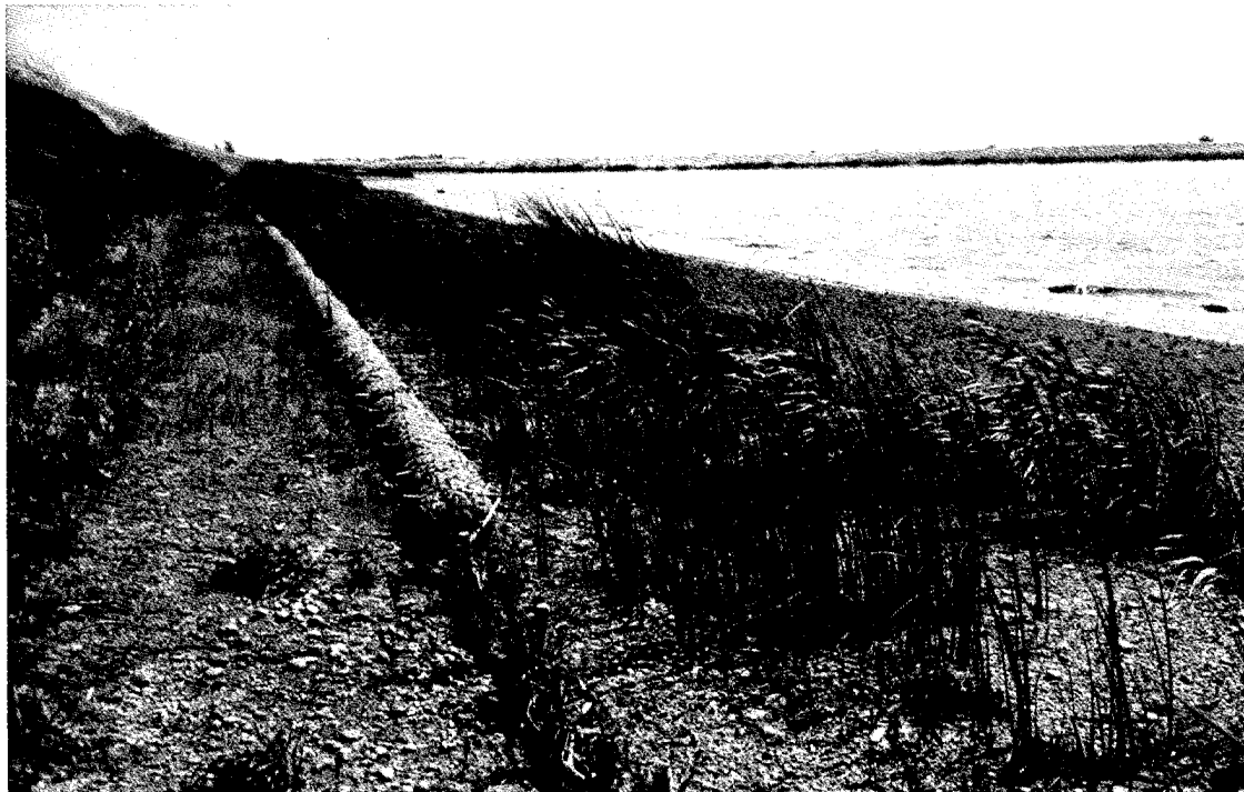
Figure F8. Erosion control measures implemented on the west side of the site above the east breach (High summer winds, long fetch, and waves resulted in significant erosion the first year. After implementation of erosion control measures in 1993 and 1994, emergent vegetation and planted woody vegetation began to stabilize the shoreline and levees.)
