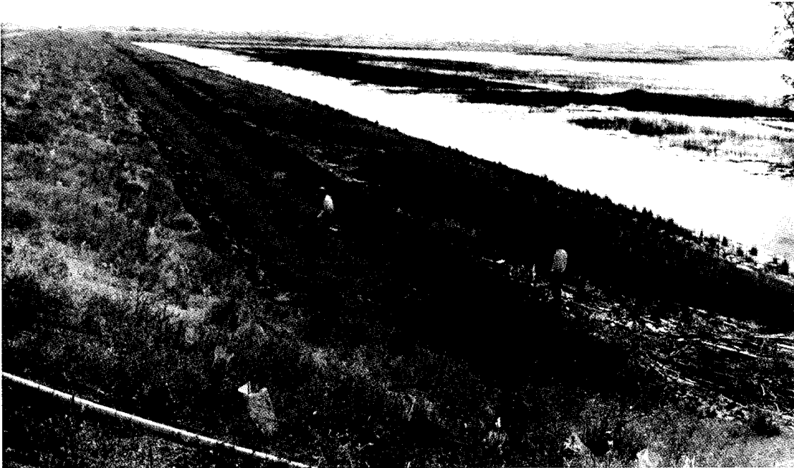
Northwest corner facing east. Cross levee plantings
