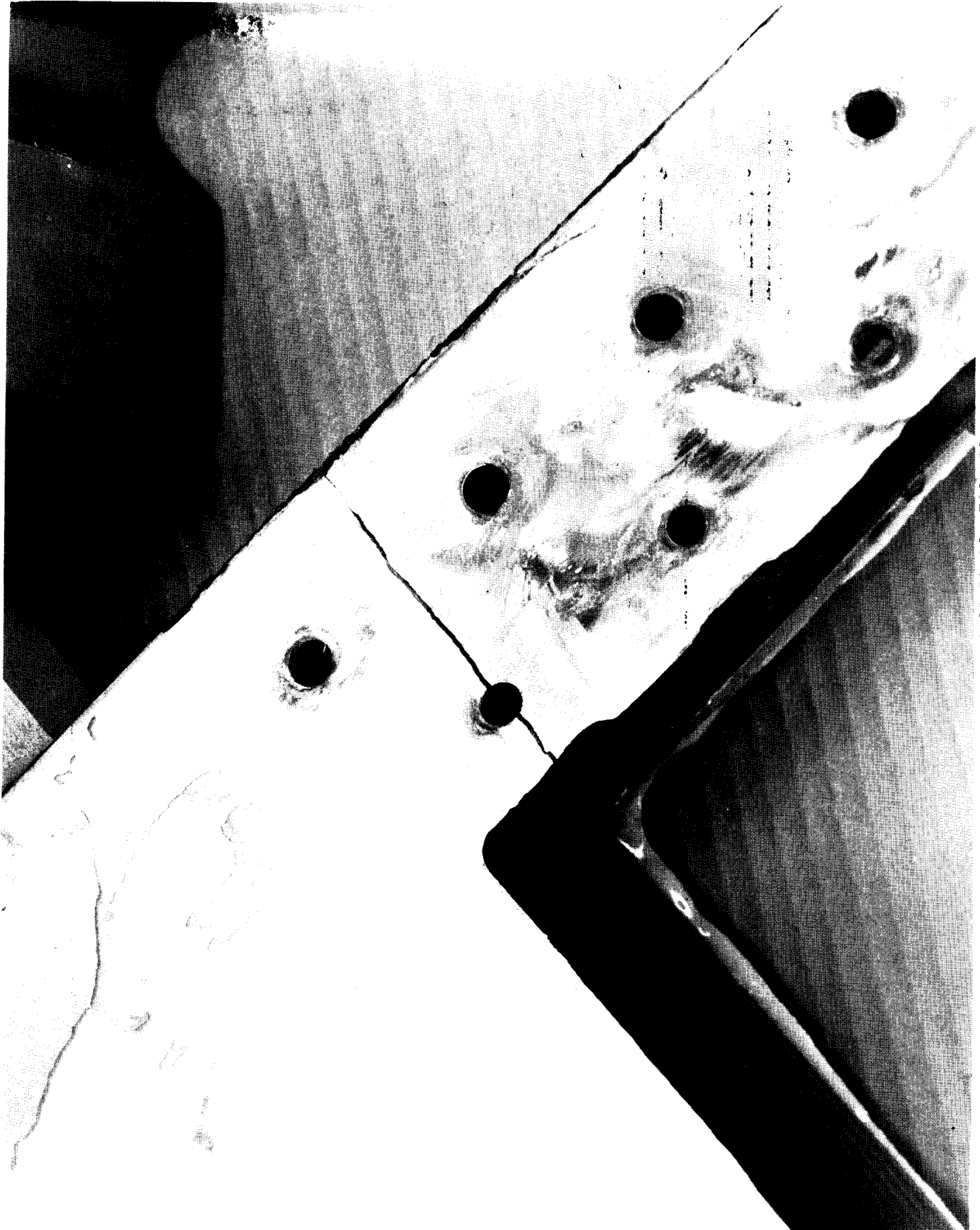
FIGURE 5-9 TITANIUM CLOSURE RIB FAILURE
