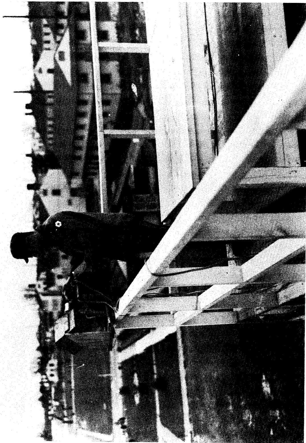
6. Adjusting pyranometers which are mounted to measure the radiation on a surface facing east at  $45^{\circ}$ . These instruments were used for some time before the recording thermocouples were installed on the tower.
