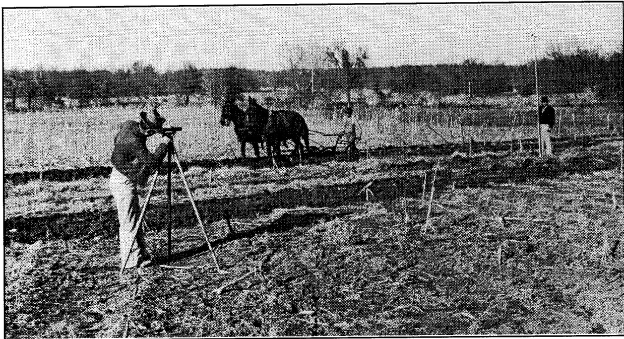
Figure 44. Establishing Terrace Lines
