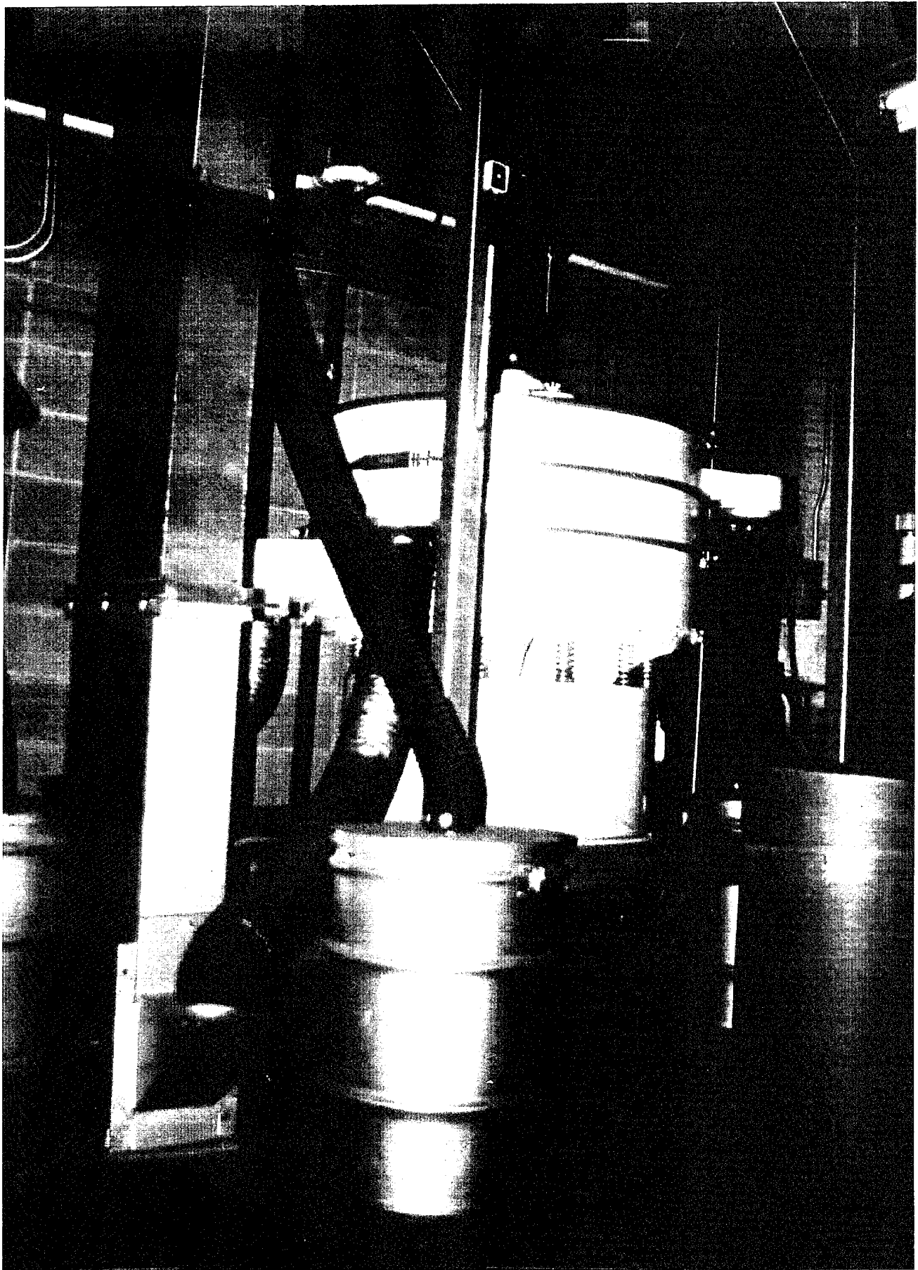
PMB media separation storage and air handling components at AVCRAD
