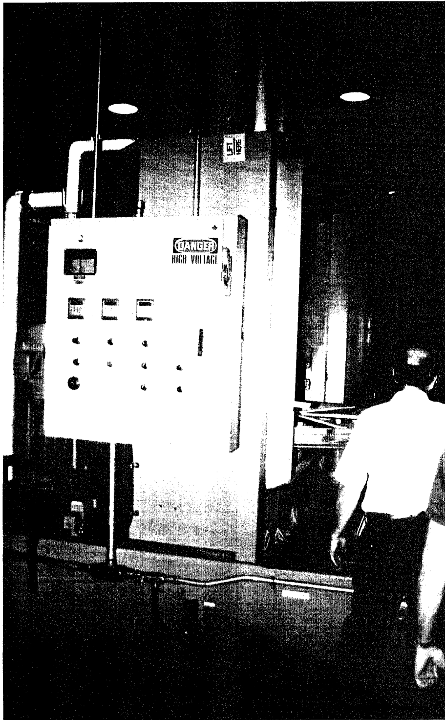
The control panel on the left side of a spay washer at SAEP
