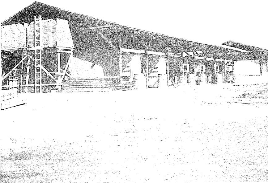
FIGURE 98.—Quartermaster refrigerated storage point on Tinian, 1945. Note the protective roof and the water storage tanks.
