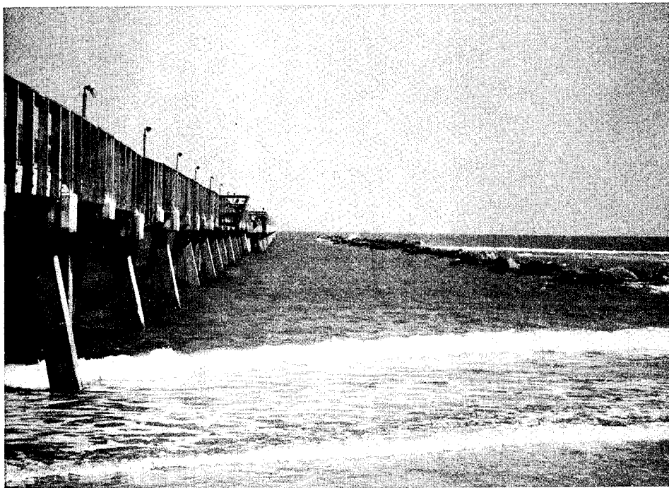
b. Looking east
