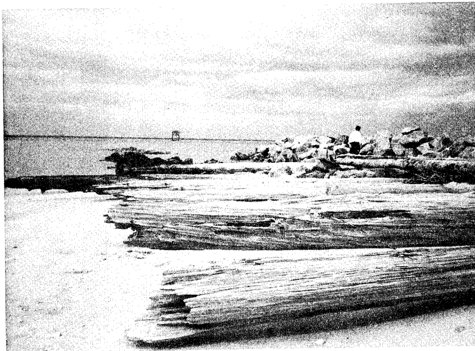
Figure G42. Jetty, looking south, January 1992, Amelia Island
