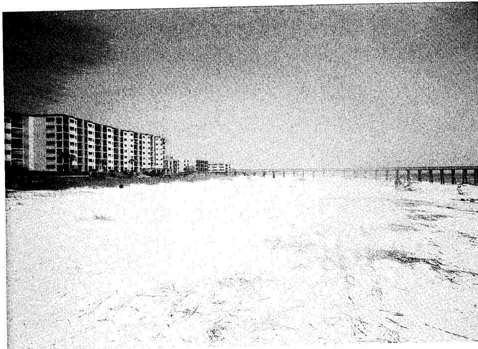
a. Looking north, including development
