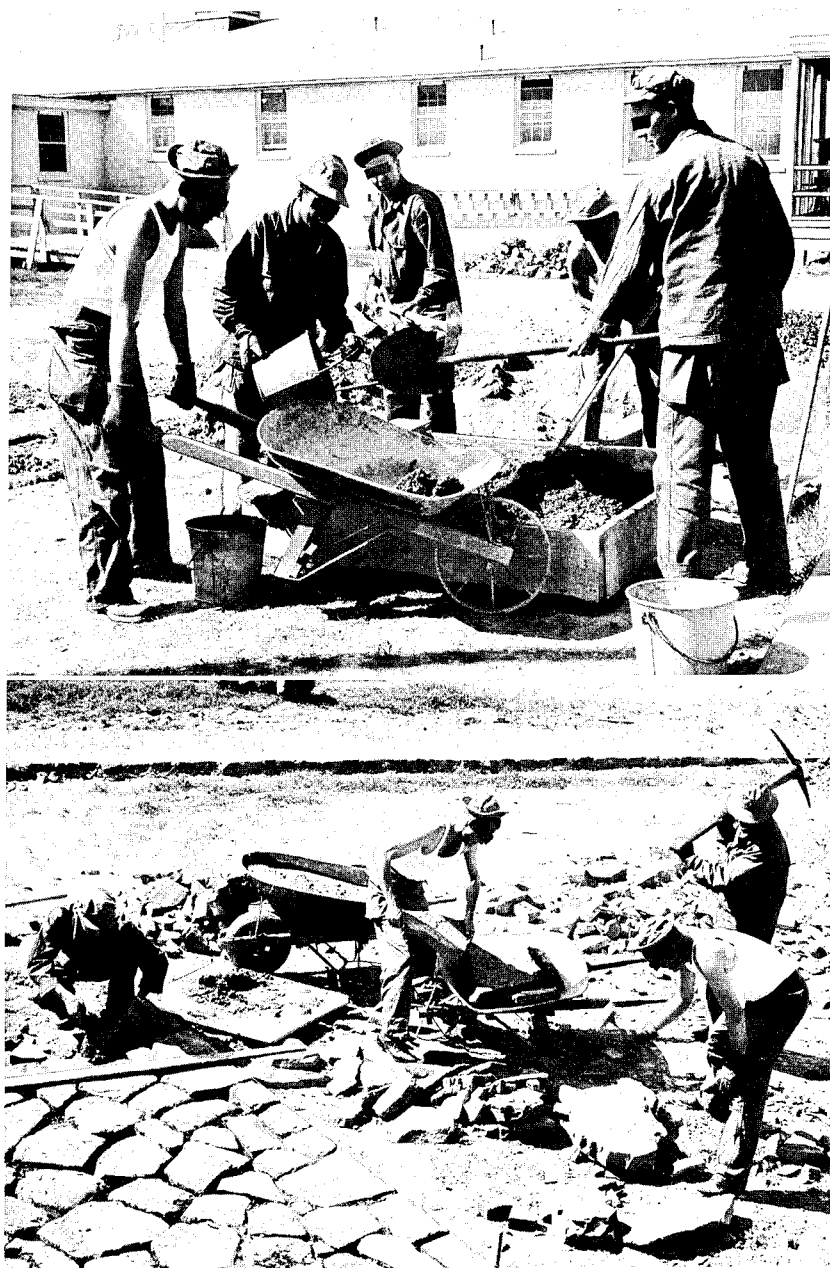
FIGURE 80—Industrial therapy providing socialization and constructive activity which benefits both the hospital and the patients. (Top) Mixing concrete. (Bottom) Setting a natural stone walk. (U.S. Army photographs.)
