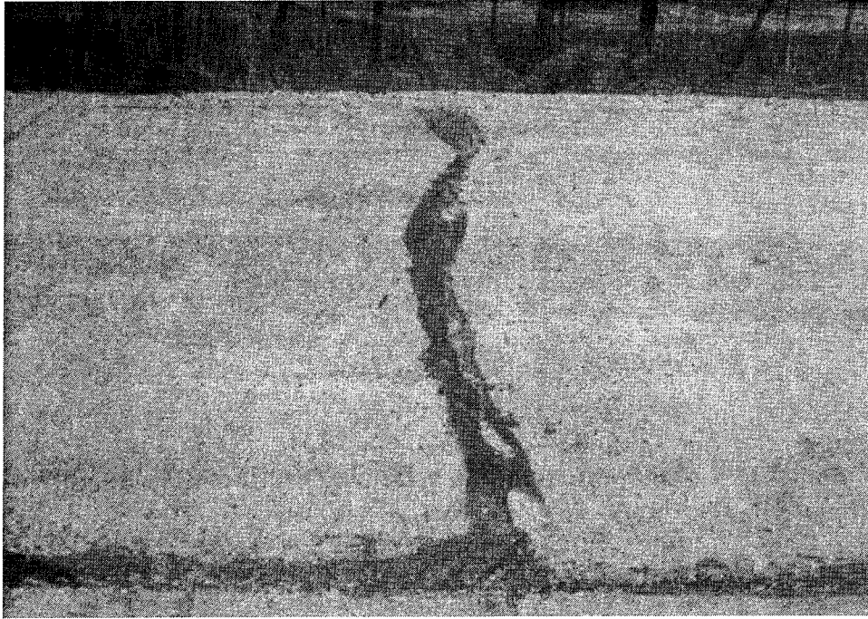
Photo F2. Asphalt patched crack (Lane II)
