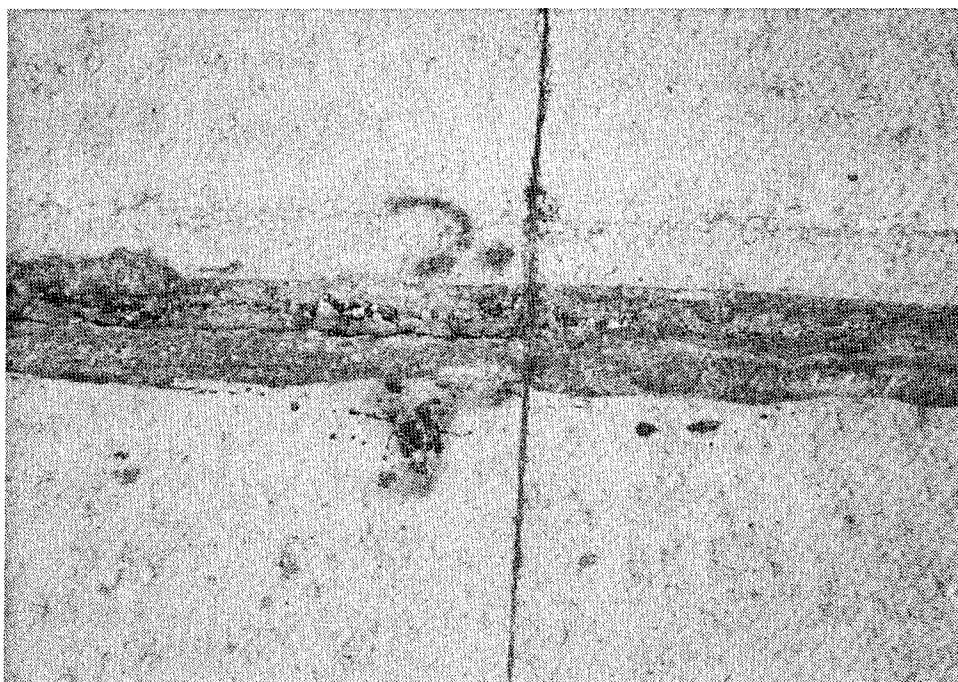
Photo A10. Close up of jointing, Lane II/dry-cut/background,Lane I/wet-cut/foreground
