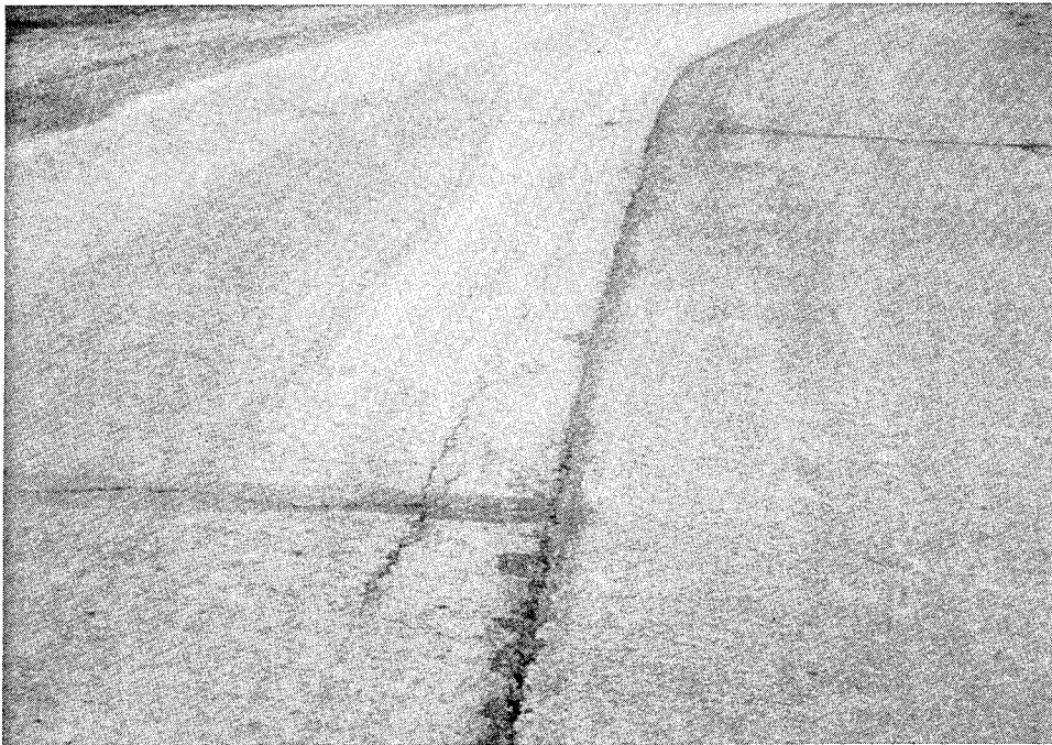
Photo F3. Longitudinal crack in Lane II 1-1/2 ft offset from longitudinal construction joint in the curve
