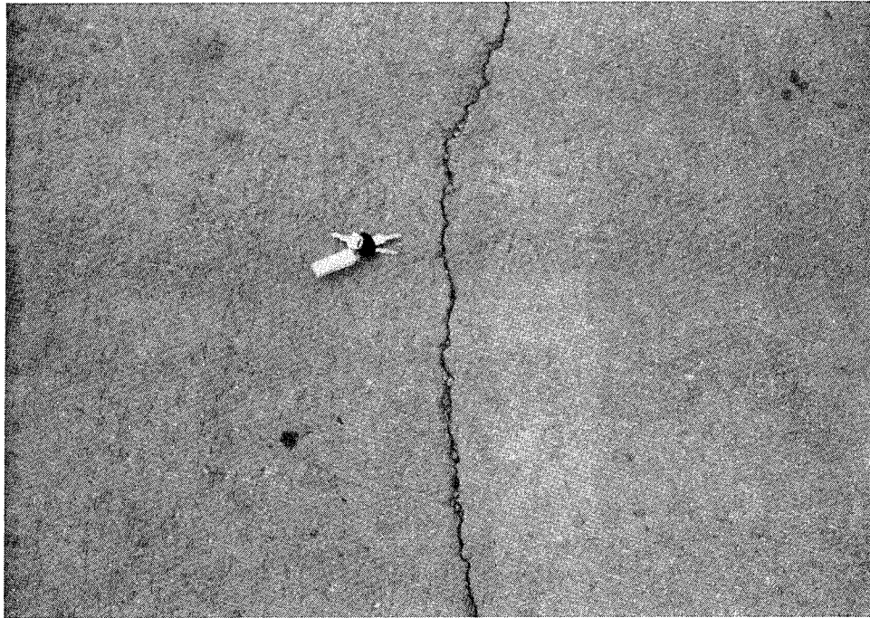
Photo F6. Typical transverse crack
