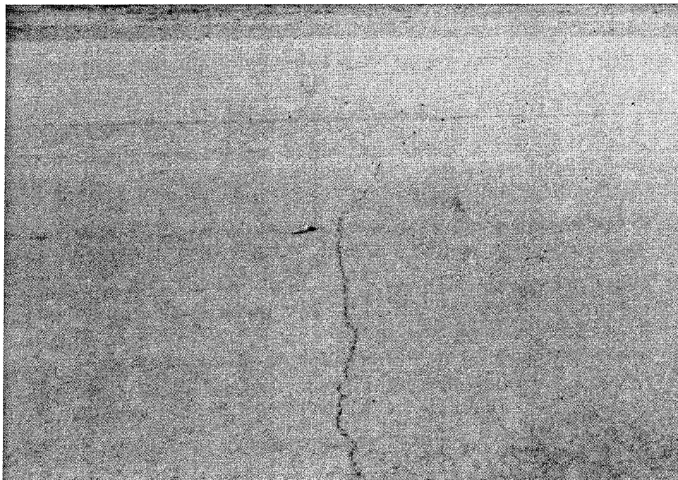
Photo F7. Transverse crack running through both lanes
