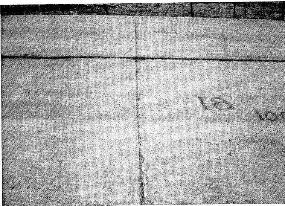
Photo A9. Transverse joint crossing both lanes, Lane 1 in foreground
