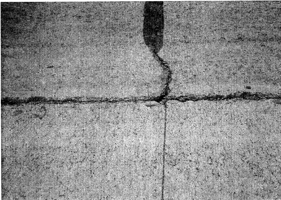
Photo F1. Sealed crack (Lane I) opposite a transverse joint (Lane II)
