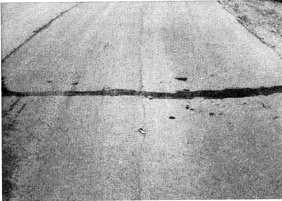
Photo F4. Sealed transverse crack with longitudinal crack centerline crack (Lane I)
