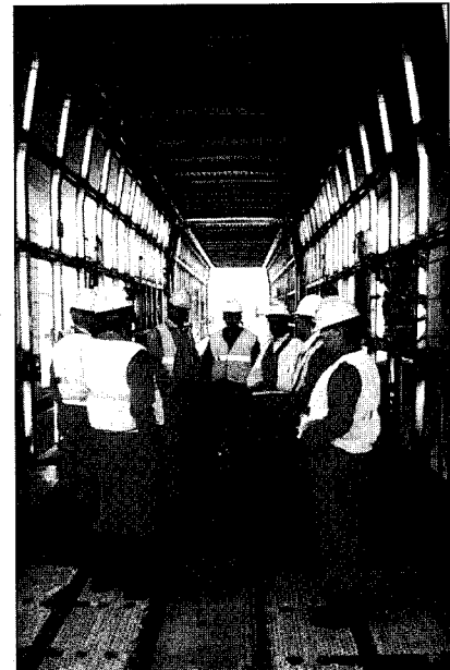
Task force members tour Channel Tunnel construction site and work in progress.
