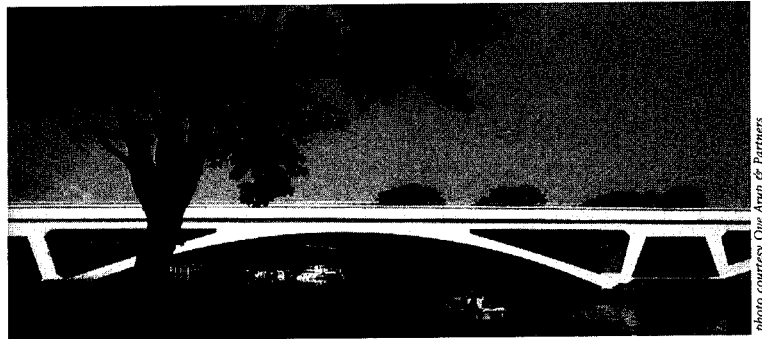
The superstructure of the second bridge at Runnymede, designed by Ove Arup & Partners, consists of four balanced frames of prestressed concrete that were cast as half frames on the bank and then slid into their final positions.
