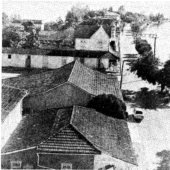
Buildings of stucco-coated brick or masonry are common in the towns of Cuba. Most are single story and have tile floors, and tile or metal roofs.
