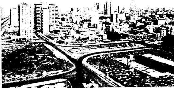
Reinforced concrete and masonry buildings are prevalent in Havana City.
