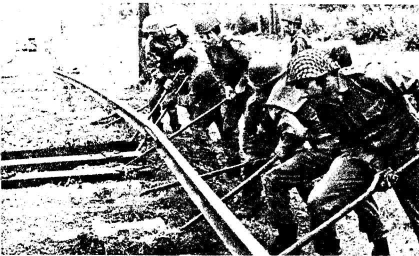
A reserve railroad unit repairs some railroad tracks. The unit is subordinate to MINFAR's Rear Services Headquarters.
