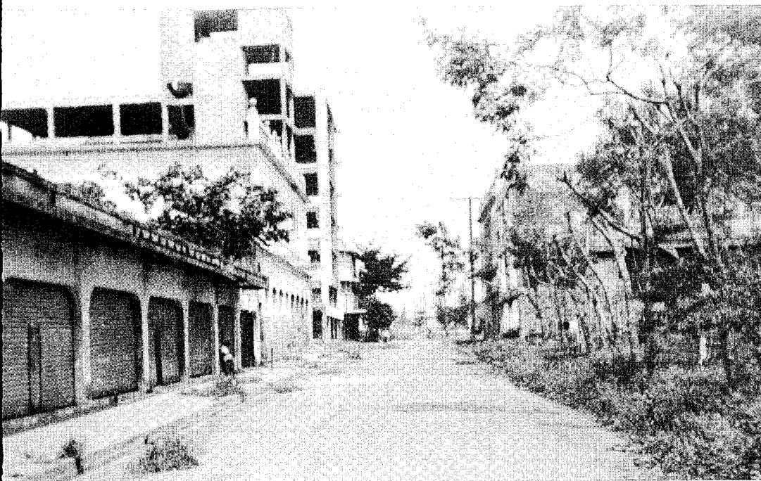
Many buildings in downtown Managua, damaged in the 1972 earthquake, remained unrepaired in 1993. Courtesy Edmundo Flores
