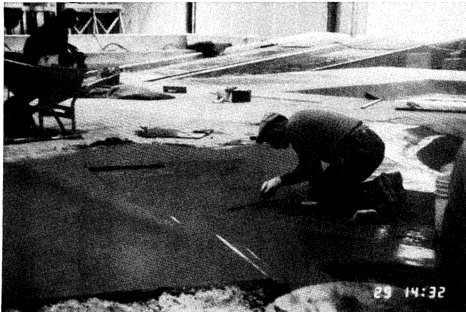
Figure 6. Construction crew working on north end of marina
