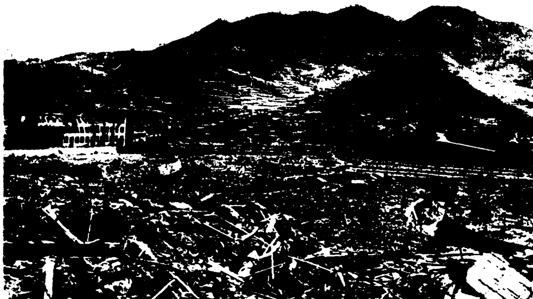
FIGURE 305.—View of Nagasaki 6 weeks after bombing, showing Roman Catholic Church that escaped heavy casualties because Mass had ended an hour earlier. Only parts of heavy brick walls still stand. Boxlike structure seen at bottom of hill to the left is the cupola. In far left is a school, whose upper story shows a slanting displacement. Building was used for industrial purposes at time of bombing, and no data could be secured concerning casualties among the work force. Shacks in foreground were constructed after bombing. Kindling in foreground is in an unburned area. The ground between this area and background is covered with ashes of houses, in which are skeletons consumed by fire within them.
