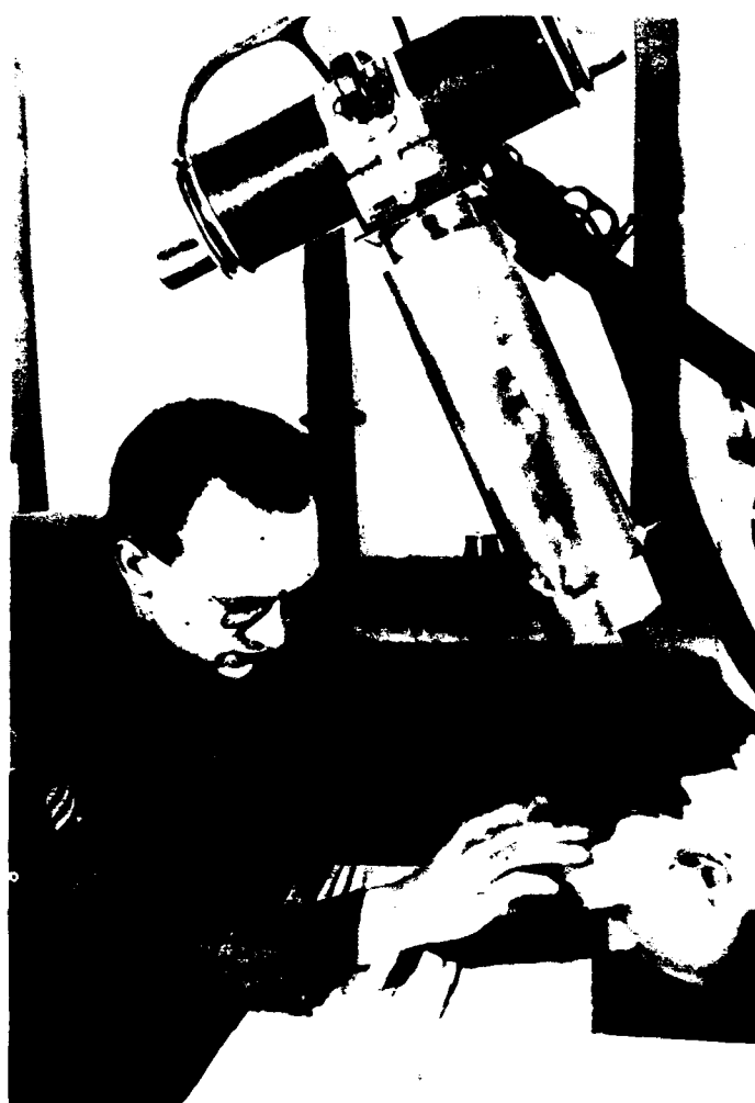
FIGURE 77.—Extension cylinder, heavy but efficient, constructed from shell casings and attached to Picker field unit. Note also mahogany plywood tabletop. 36th General Hospital, Caserta, Italy.
