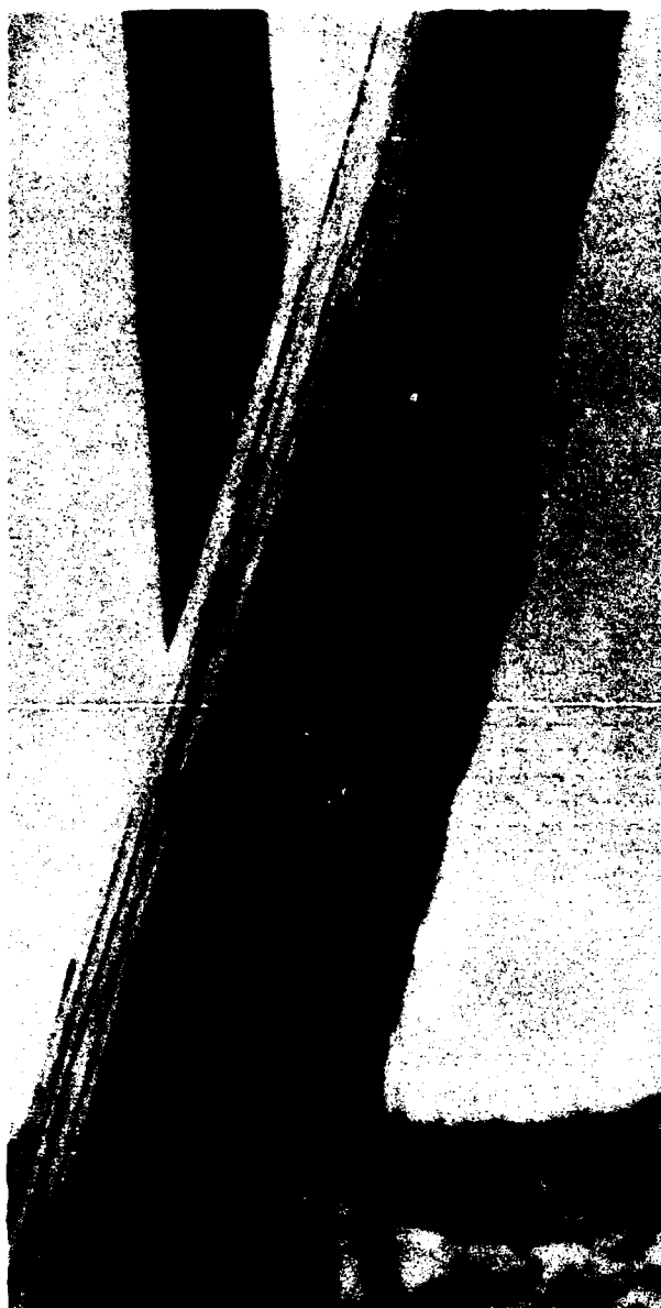
FIGURE 298.—Telephone post at considerable distance south of zero point, Nagasaki, charred on side toward detonation. The fire apparently continued to burn for some time after the blast. Note that radiation in this picture has come from the side rather than from above, as in figure 296. Intact pole is a postdetonation replacement.
