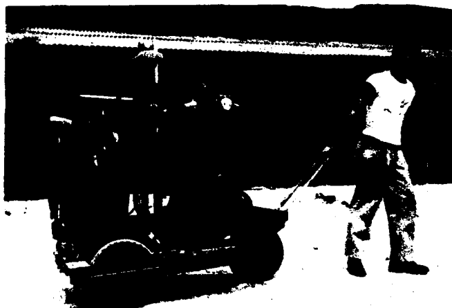
FIGURE 212.—Portable X-ray unit and power generator equipped with airplane tires, 9th General Hospital, Goodenough Island, 1944. Without some such equipment, to aid in getting the X-ray machine to the patient's bedside through mud and muck or over rough ground, a portable unit was not portable.
