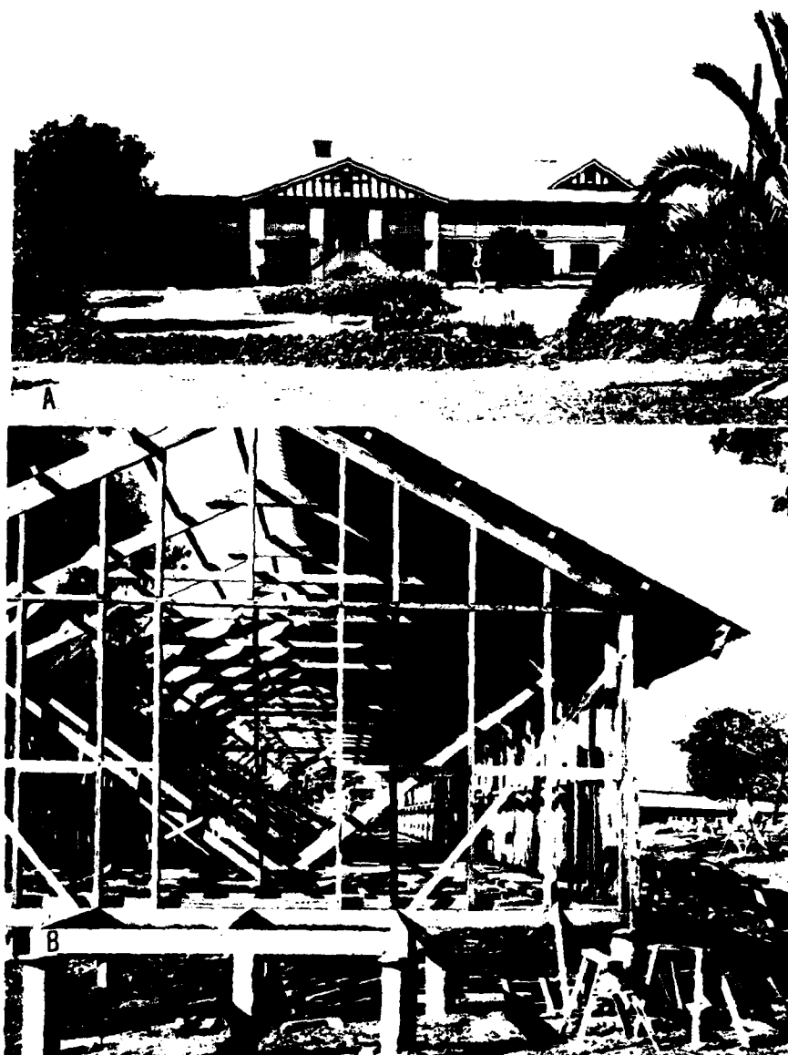
FIGURE 198.—Gatton College, Queensland, Australia, location of 105th General Hospital. A. College building. B. Additional ward under construction, November 1942. Note pie tins used on top of pilings, to prevent destruction by termites.
