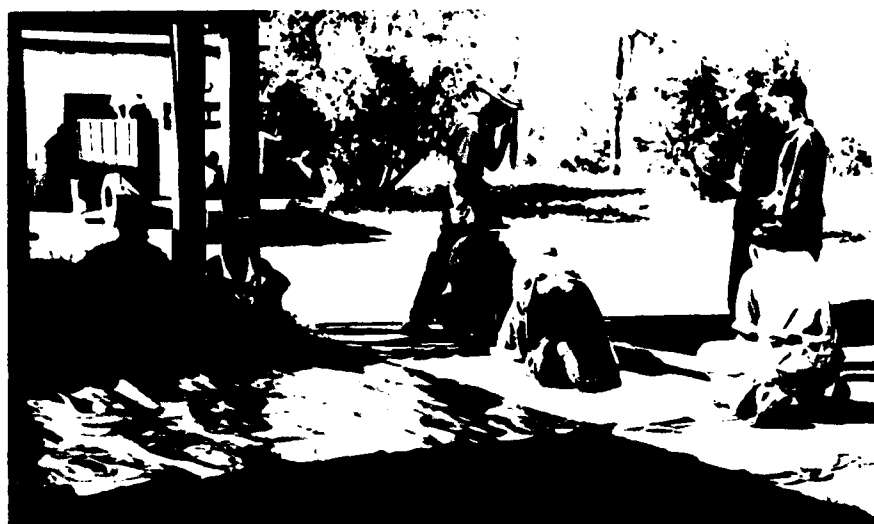
FIGURE 194.—Unrolling sheet lead to be used for walls of X-ray department of 105th General Hospital at Gatton, Australia, January 1943.
