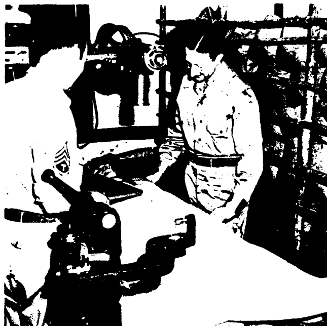
FIGURE 240.—X-ray room, 20th General Hospital. Note sandbags, held in place by bamboo poles, for protection of personnel against radiation.
