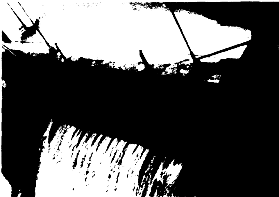
Figure 12. Riveted vertical-lift gate at Bankhead Dam
