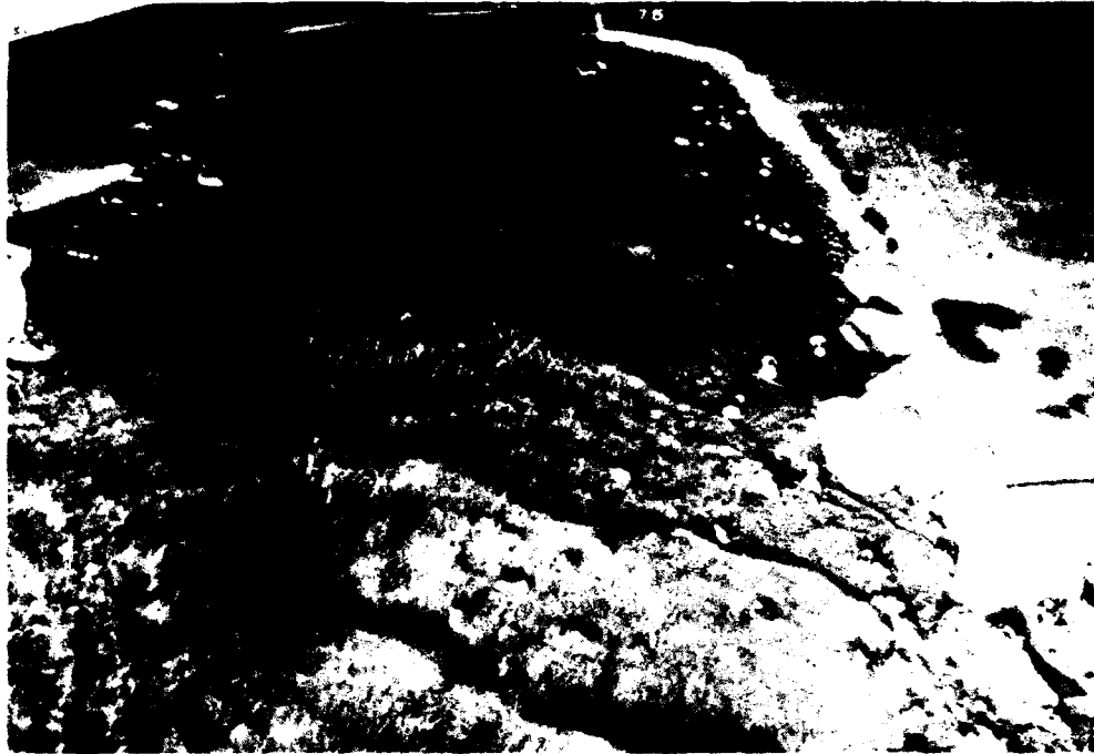
Photo 51. Riverine sediment tracer patterns for existing conditions; 13-sec, 14-ft waves from west-northwest; swl = 0.0 ft, 20,000-cfs river discharge
