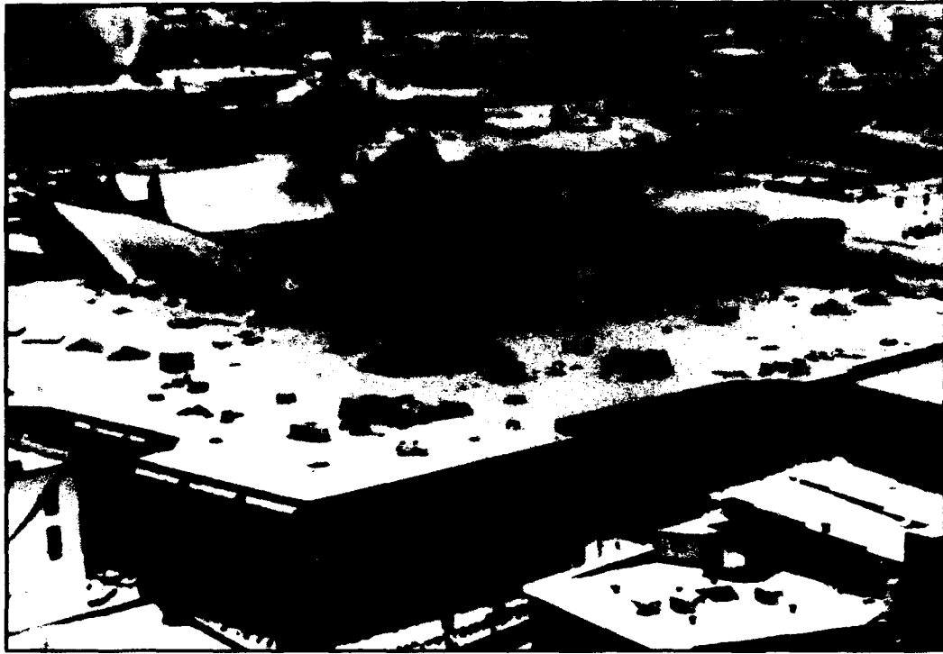
Figure 7.7. The Hartford Coliseum after its roof collapsed. The contorted corners of the space frame are visible above the roof level. (AP/Wide World Photos)
