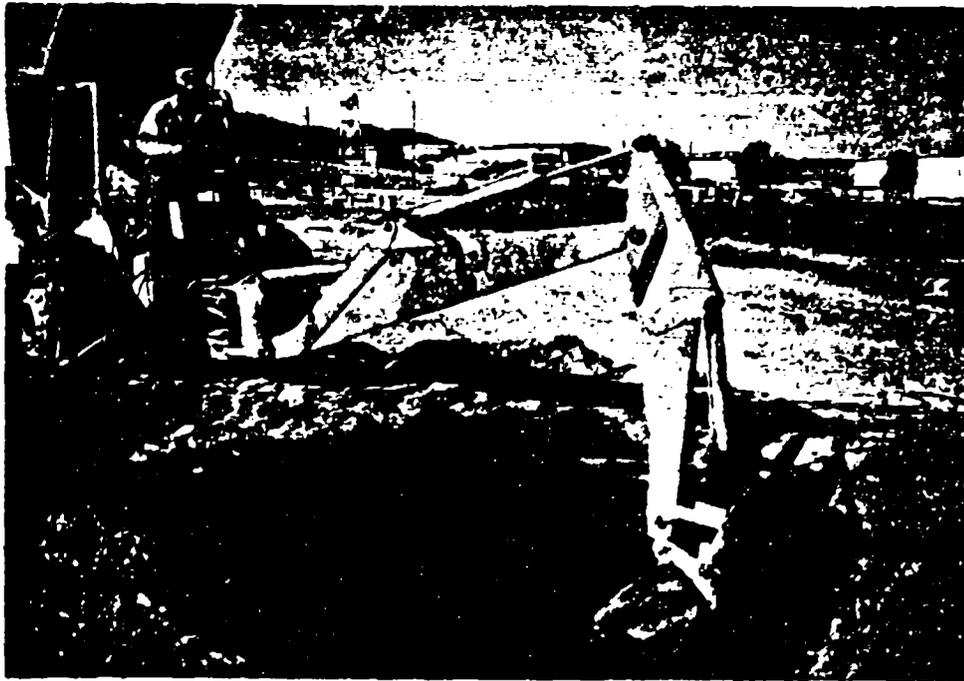
Figure 3.17 Removal of Sand with Backhoe.
