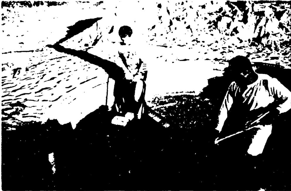
Figure 3.14 Vibratory Compaction of Lifts
