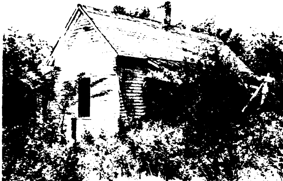
House, viewer facing Northwest
