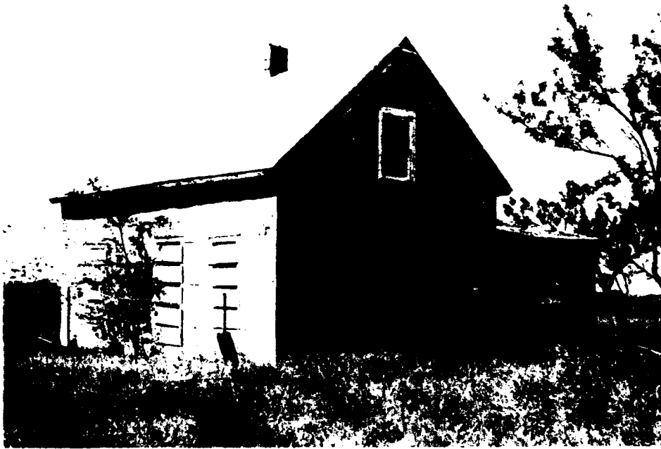
Log cabin house, viewer facing Southwest
