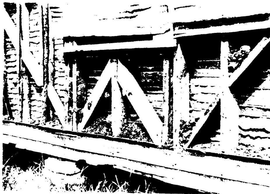
Detail of structure on west side of house
