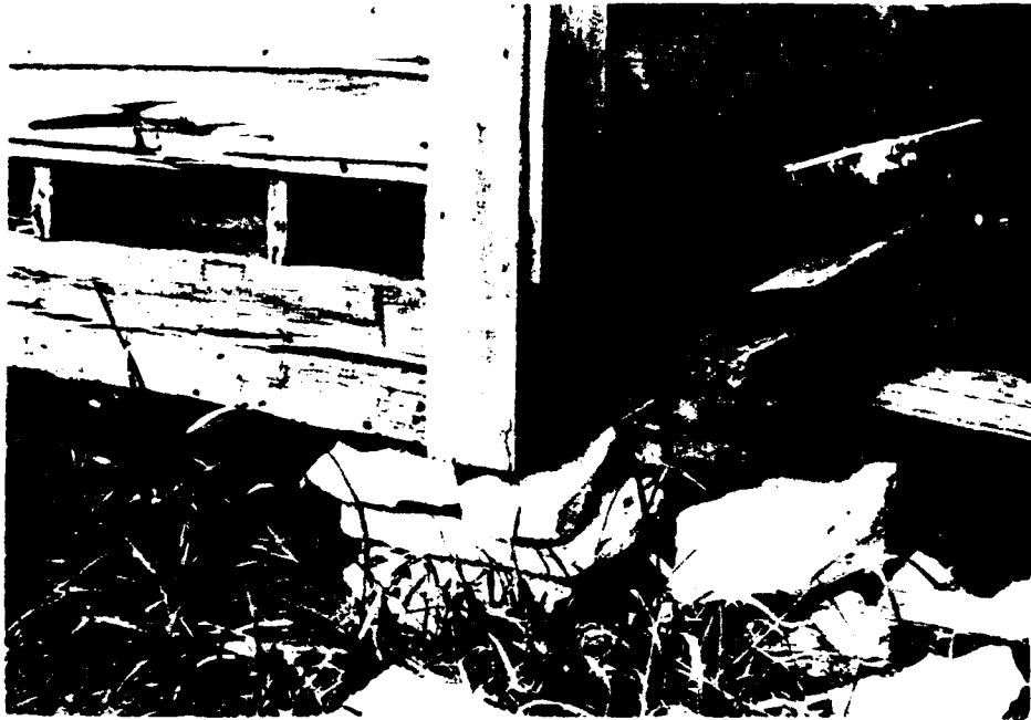
Detail of Southwest corner of house, showing field stone corner supports, hand-hewn beams
