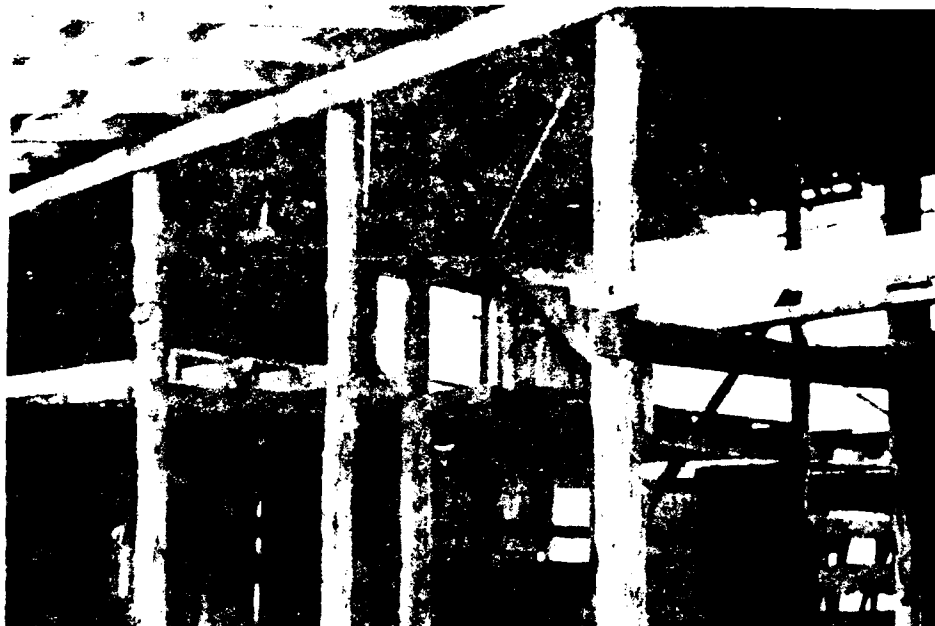
Interior of barn, showing pole-type construction
