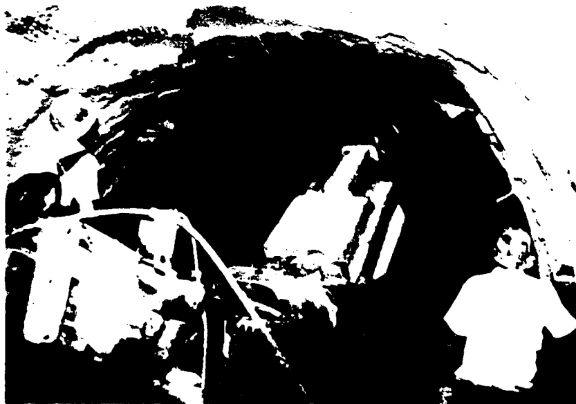
Roadheader excavation beneath spiling crown support in tail tunnel. View at 80-foot length of excavation. Shape is 14-foot wide horseshoe.
