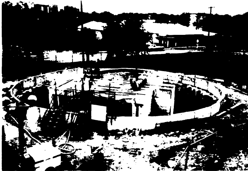
View SW at concrete surface structure of inlet shaft. Excavation to 68-foot depth, elev 590.
