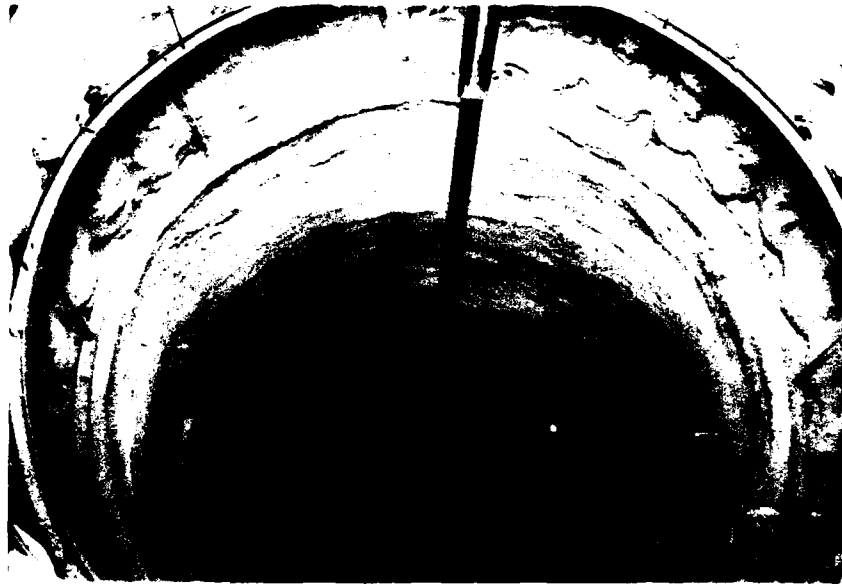
Drilling 22.0-foot diameter shaft to provide access for top heading tunnel excavations. Shaft at Sta 23+63.
