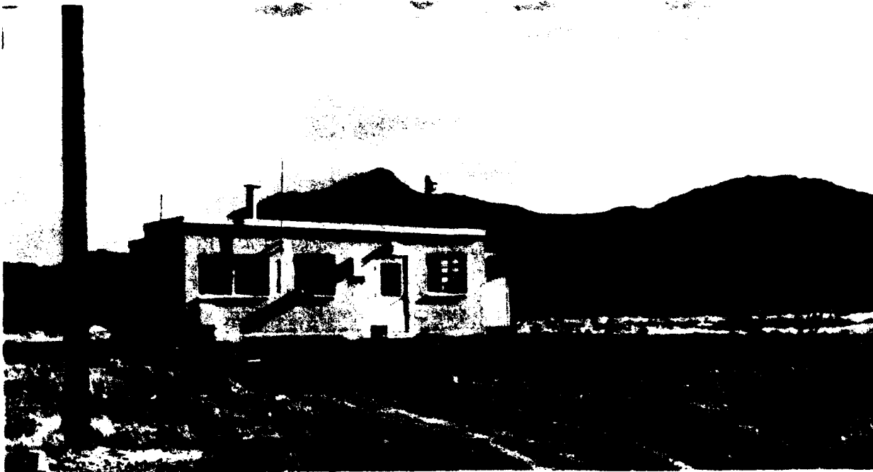
Figure 6. The Tower Grid Command Post (CP) at Dugway Proving Ground. (Photograph by the U.S. Army Dugway Proving Ground Technical Systems Branch.)
