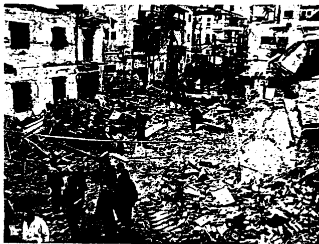
Figure 1 - Structures damaged by missile attack
