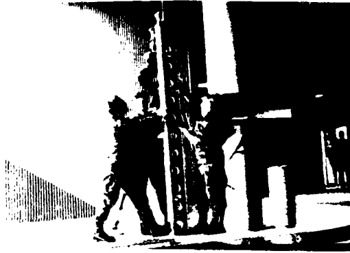
Figure 9. FOAL EAGLE - Nearly Completed Column Replacement Repair.
