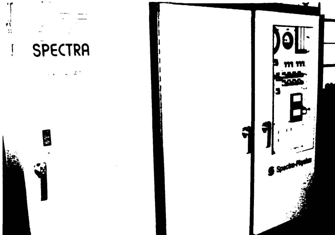
Figure 11. Power supply cabinet for laser.
