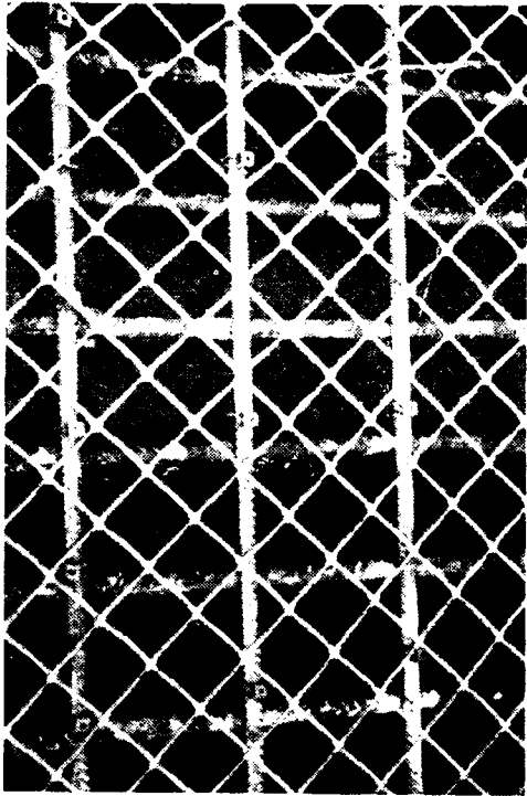
FIGURE 1 Plastic spacer mesh and push-on fasteners on rebar ready for placement of activated titanium anode mesh.
