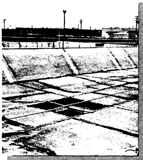
Site 42/PRL 68 Area (IWTP Blending Ponds)
