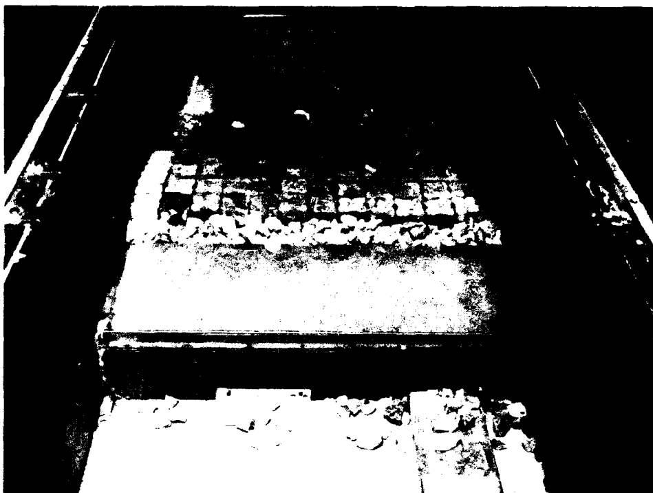
Photo 37. Land-side view of Plan 7R after wave attack
