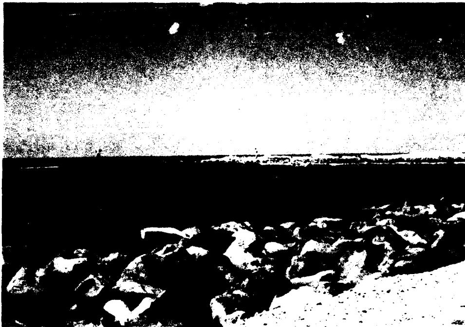
Figure 83. Rubble-mound wave absorber
