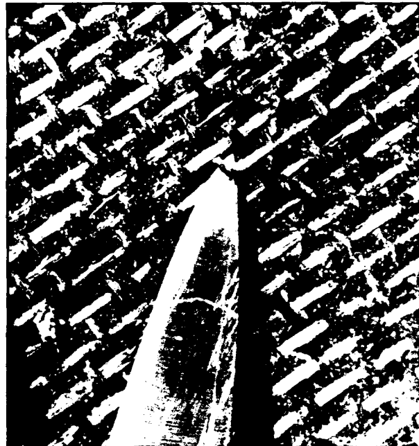
MDH1 <High Severity> Scrim completely exposed
