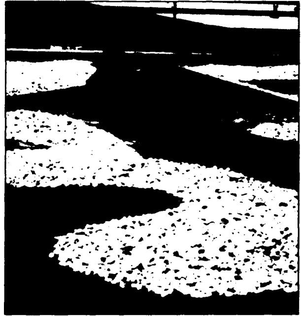
SSH4 <High Severity> Ballasted system, bare area more than 100 sq ft
