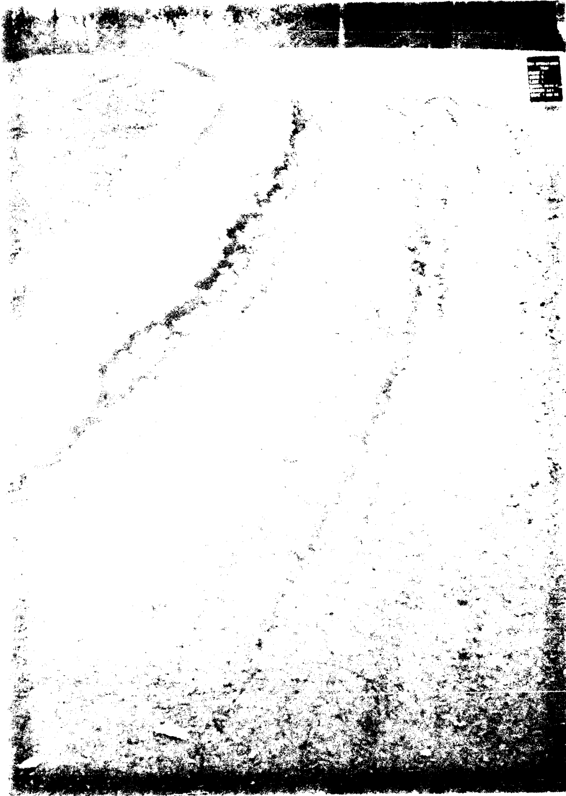
Photo 18. Item 5, wheel path, high-severity rutting and cracking in a localized area
