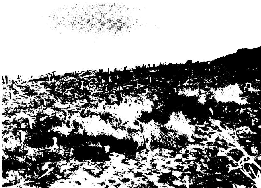
Figure 25. Baker Bay project site, barren wattles after three inundations (lower right and middle left). Note matting in center is heavily invaded and stabilized by reed canarygrass
