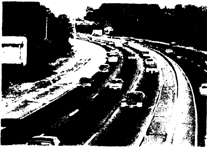
LEVEL OF SERVICE B
