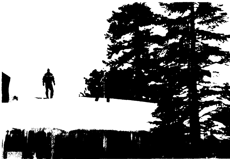
Figure 5. North-facing Eave with Ice Dam. Note ridgeline is free of snow while ice dam and southern winds build up snow on north-facing roof.
