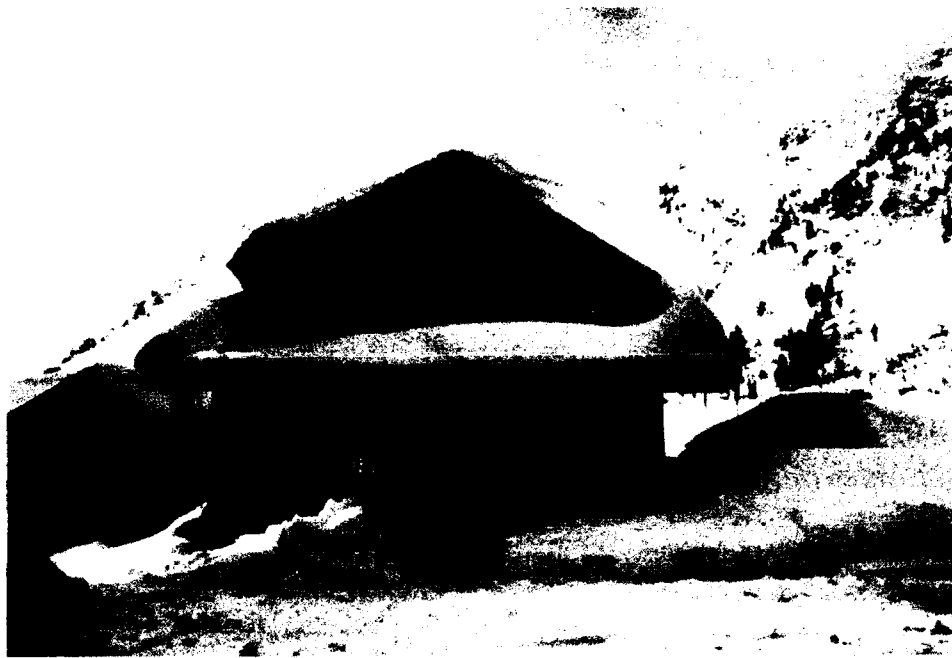
Figure 4. Unbalanced Snow Distribution. North-facing roof on right with about five times more snow than "sun-drenched" south-facing roof.
