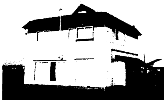
Fig. 17 House Yajirobeh constructed for roof snow to be kept on the roof (Nagaoka, built in 1988).
