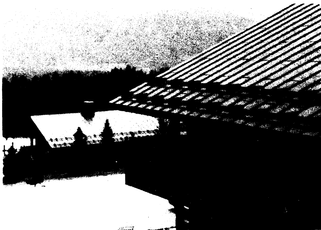
Snow guards are used to hold snow on these metal roofs in Vermont, U.S.A. (Photograph by Wayne Tobiasson.)
