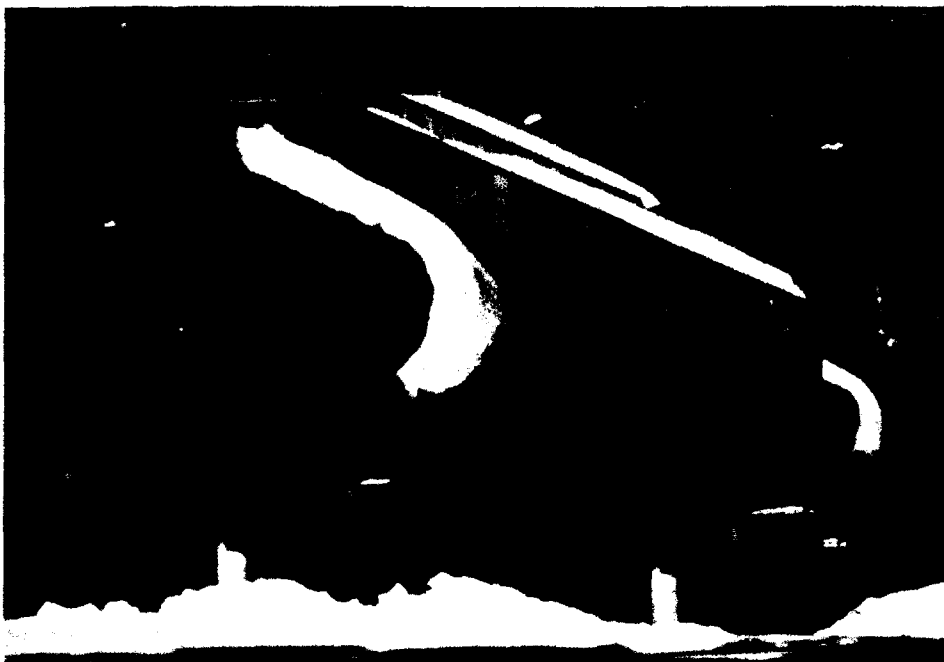
Figure 3. Cantilevered Snow/Ice Curl. Slow snow creep on a metal roof causes this type of unbalanced load.
