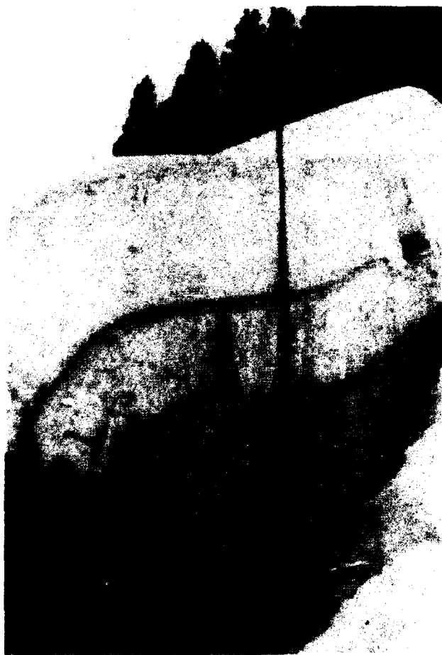
Heavy snow load on avalanche defense structures in Japan and damage that has resulted in new design criteria. (Photographs provided by Katsumi Katakawa.)
