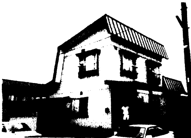
Figure 15. House designed for roof snow to slide down onto the ground with 1 m high base (Shinjo, built in 1975).
