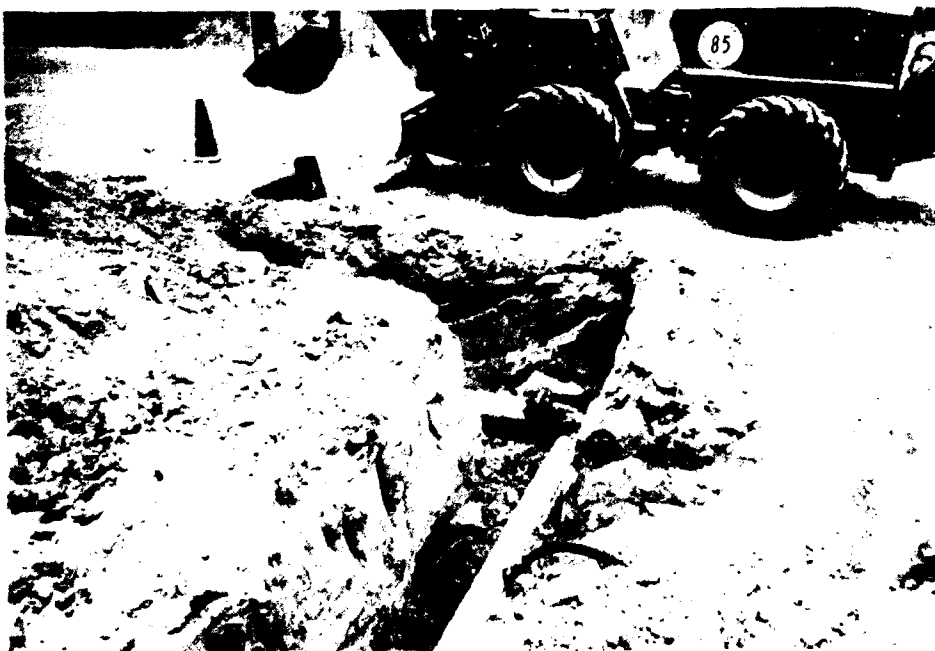
Construction of 6" Water Supply Lines
