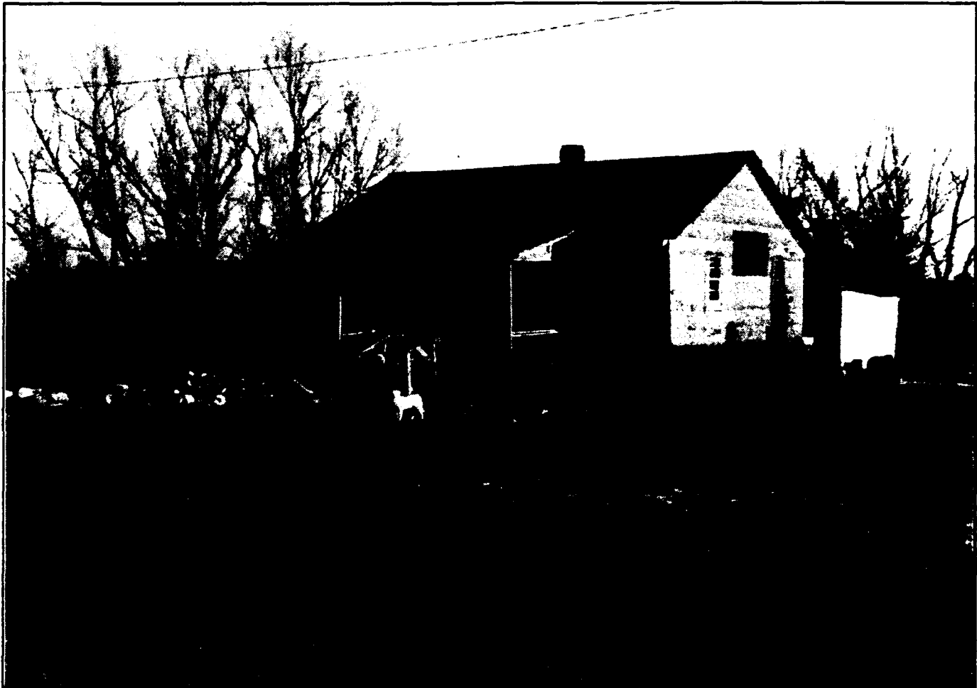
Figure 3. Photograph of Structure Moved from 3SF332.
