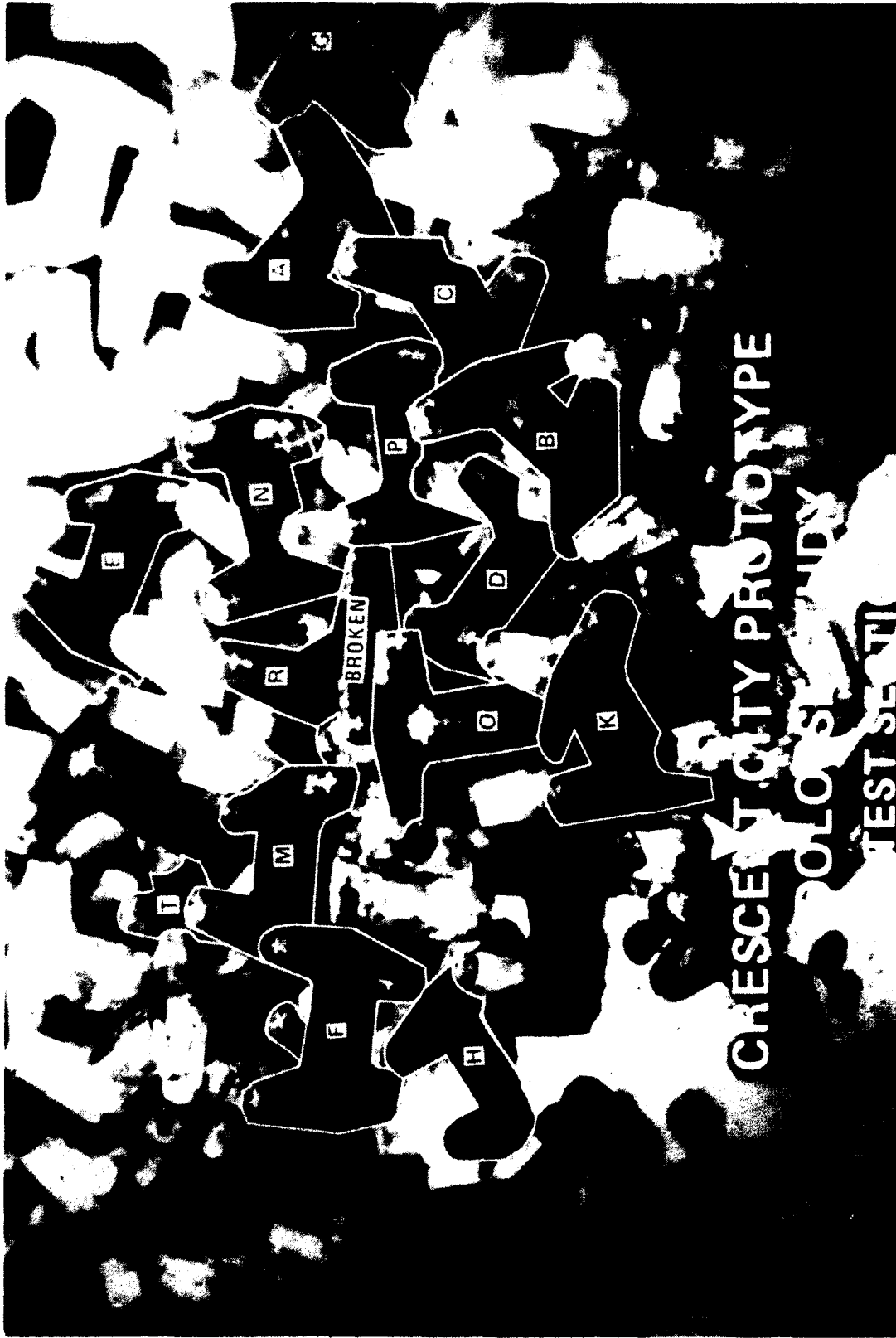
Figure 33. Aerial view of instrumented prototype dolosse on Crescent City breakwater
