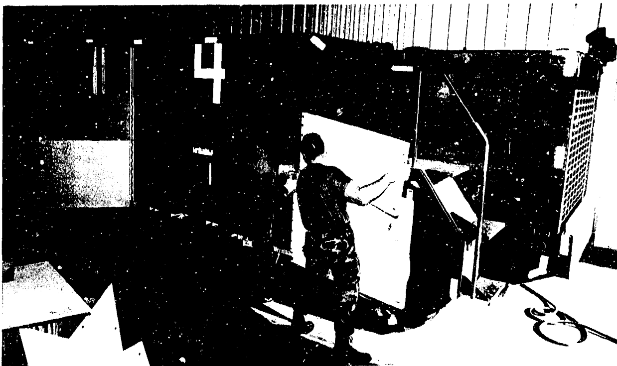
Figure 3. P-19 Armor Kit Installation
