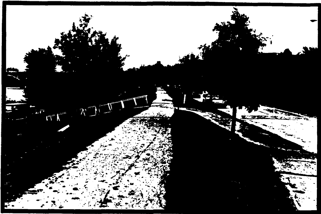
Plate 1. Bermed Sidewalk on West Side of River Drive, View to the North-Northeast. Field Date: October 8, 1992
