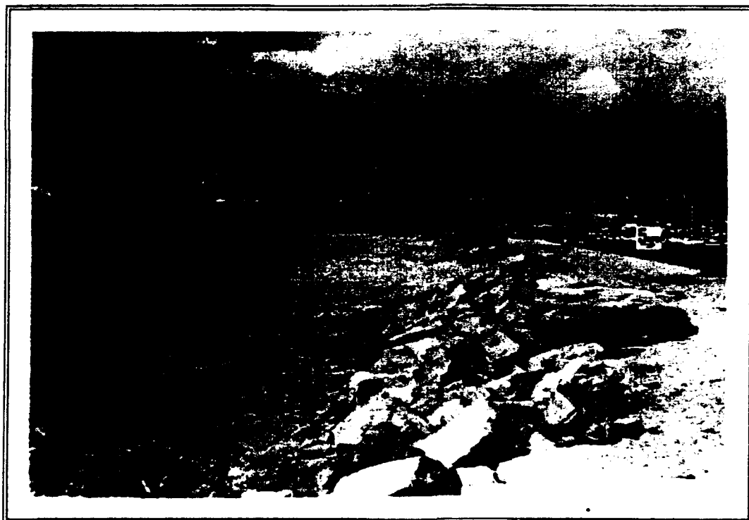
View along west side of west jetty looking north towards Santa Cruz. NOTE how sand has accumulated along the jetty.
