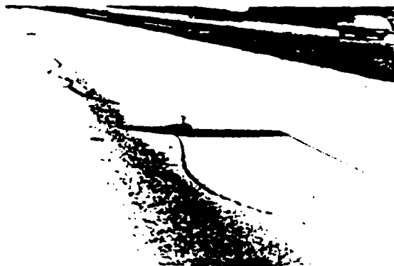
Fig. 3.2.4.2 — Meandering crack
