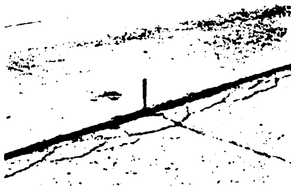
Fig. 3.2.3.8 — Lane/shoulder dropoff
