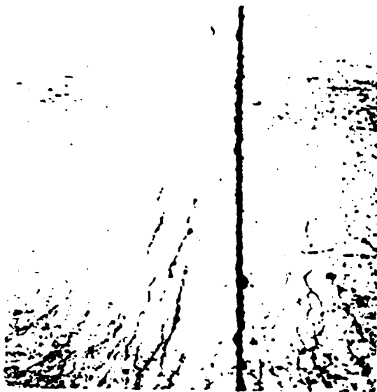
Fig. 3.2.4.4 — D-cracking
