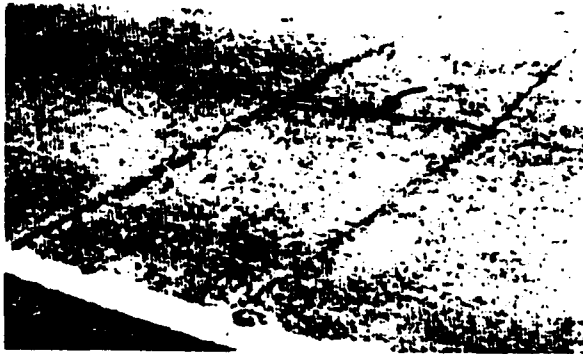
Fig. 3.2.4.8(a) — Punchout, Severity 2
