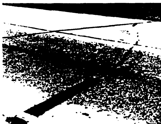
Fig. 3.2.4.6 — Diagonal crack
