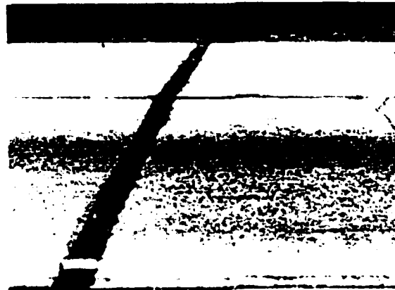
Fig. 3.2.5.2(b) — Pressure relief joint
