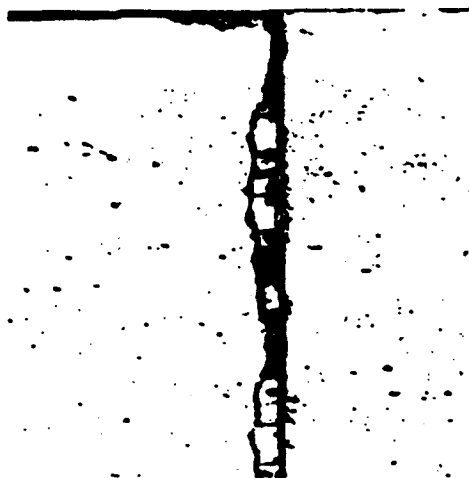
Fig. 3.2.3.9 — Joint spalling
