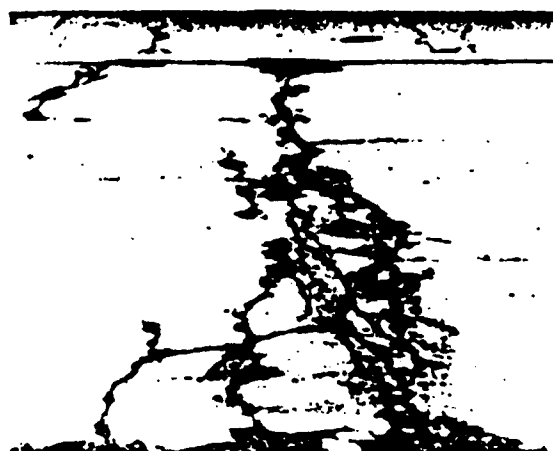
Fig. 3.2.4.5(b) — Transverse crack, multiple
