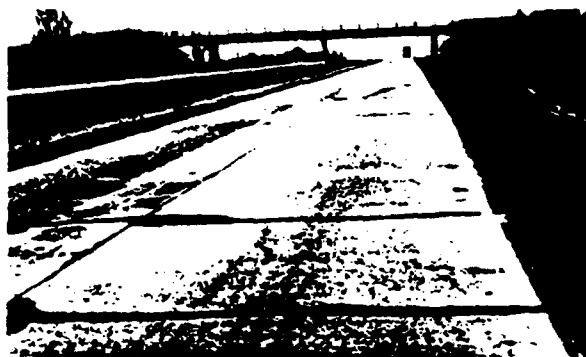
Fig. 3.2.3.5 — Joint sealant extruded
