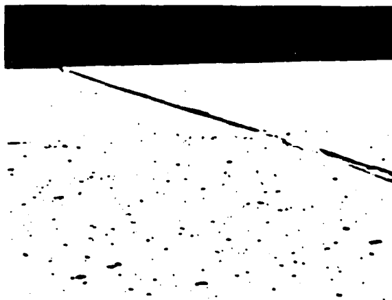
Fig. 3.2.1.2 — Aggregate pop-outs
