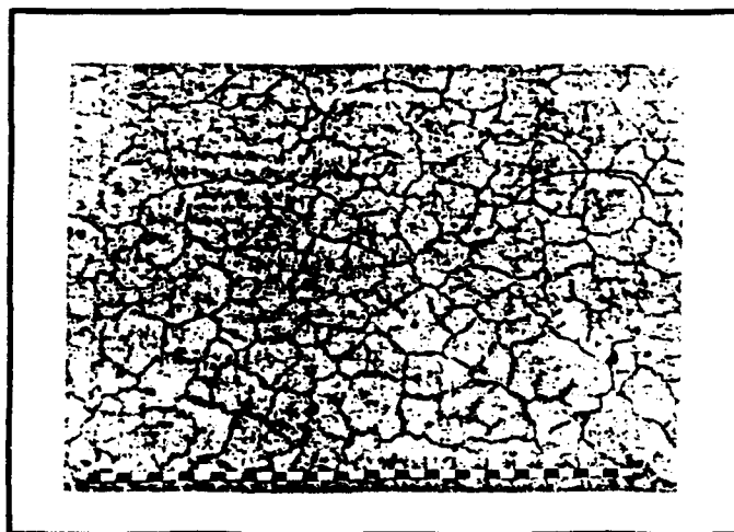
Figure 2.2 Map Cracking (Reference 4)
