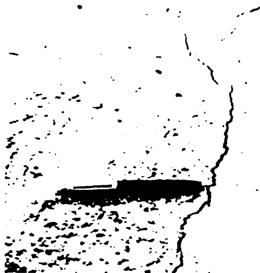
Fig. 3.2.4.10 — Plastic shrinkage cracks
