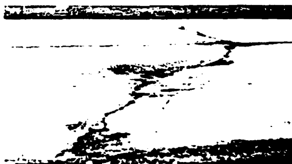
Fig. 3.2.2.3(a) — Pumping (slight)
