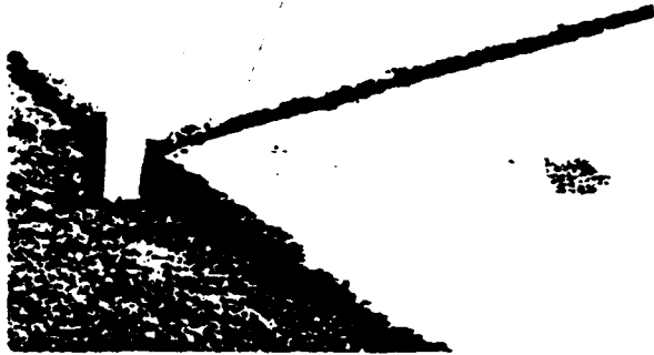
Fig. 3.2.2.1 — Faulting (stepping)
