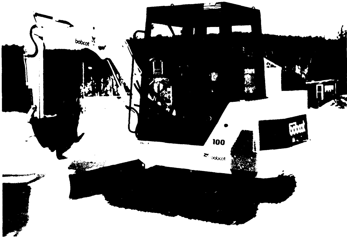
Figure 1. Bobcat 100 hydraulic excavator used for some of the digging observations (track length 81 in. [2065 mm]).
