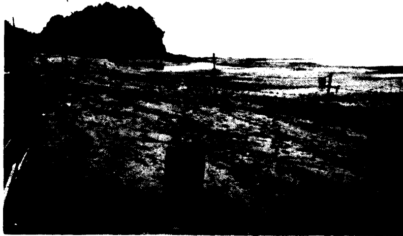
Figure 8. Completed sand cover
