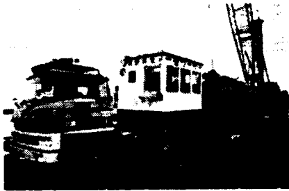
a. Transportation of components to the assembly site
