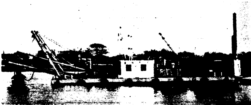
e. Assembly completed
