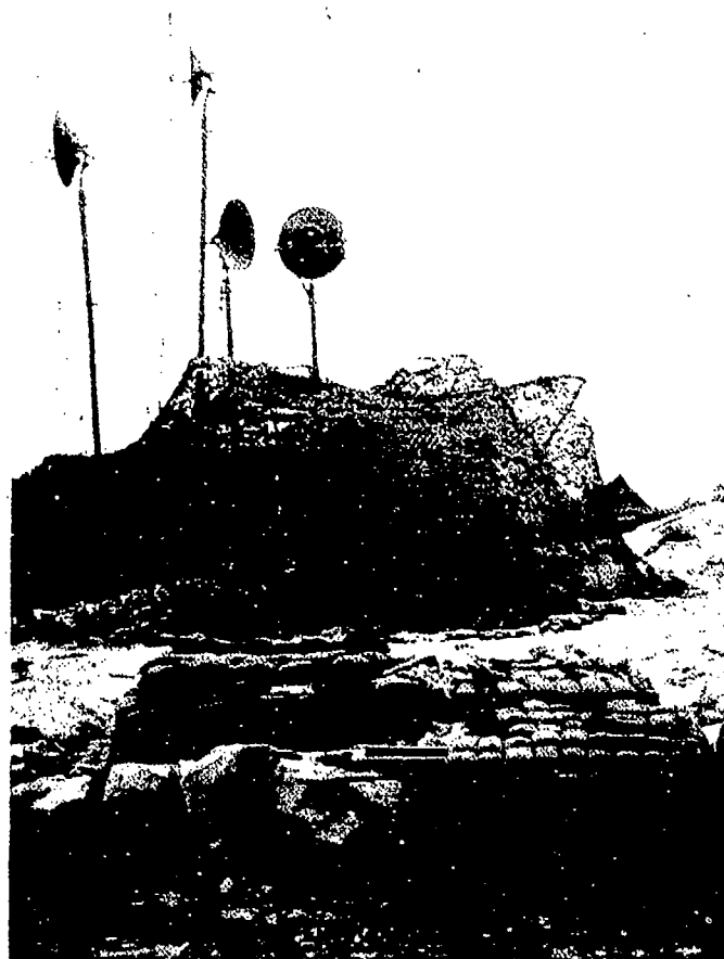
Figure K-15 Microwave Communications Relay Site Providing Communications Link Between XVIII Abn Corps and Rear Area
