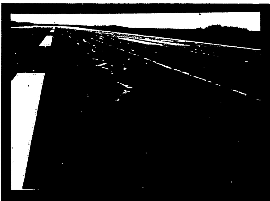
PHOTO 12: TYPICAL BLOCK CRACKING ON THE RUNWAY. CRACKS HAVE BEEN SEALED.
