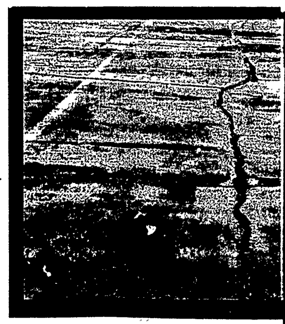
PHOTO 4 : SPALLING TRANSVERSE CRACK ON TRANSIENT APPROACH
