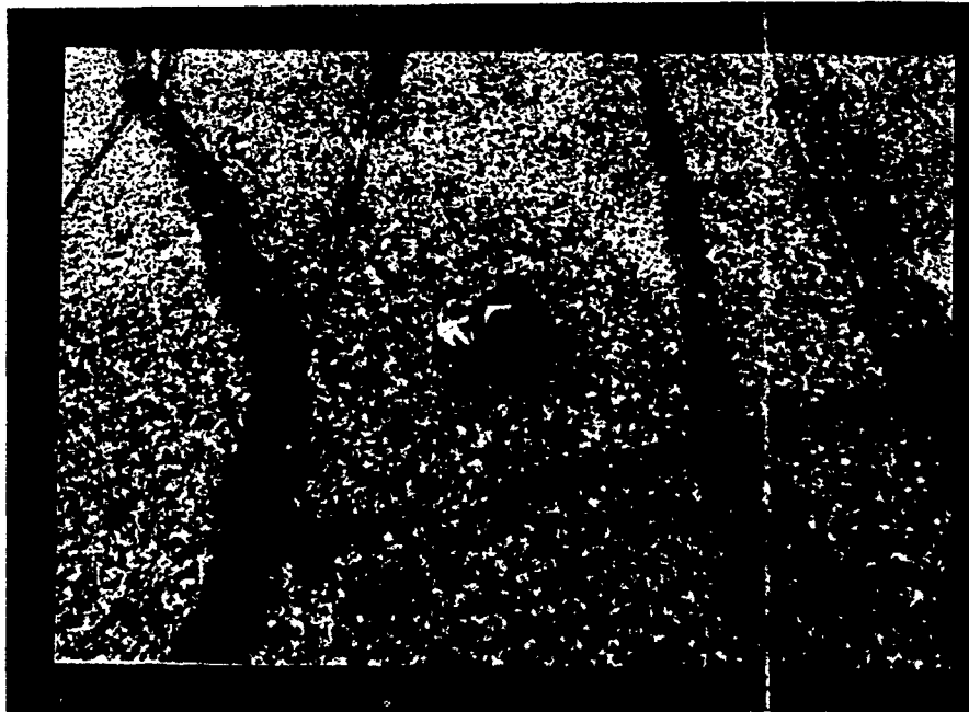
PHOTO 9 ; ERODED PCC PAVEMENT SURFACE WITH A TYPICAL LONGITUDINAL CRACK ON THE 11 END OF RUNWAY 11-29.
