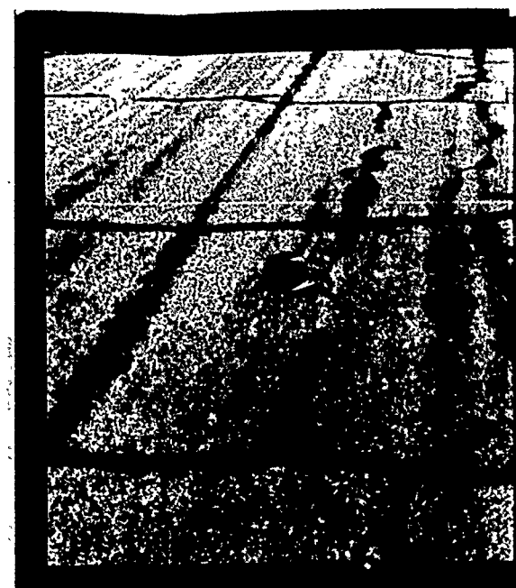
PHOTO 2 : BLOCK CRACKING, SHALLOW RUTS, AND THE BEGINNING
