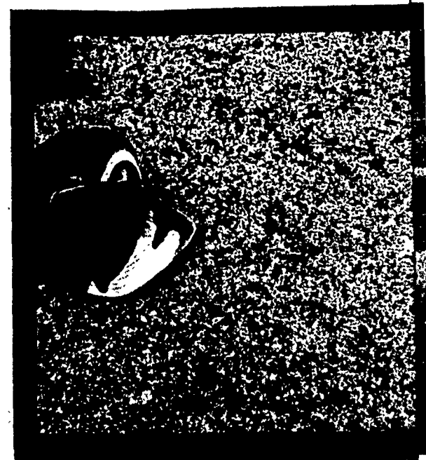
PHOTO 6 : VOIDS IN THE SURFACE OF THE PAVEMENT WHERE AGG OF TAXIWAYS 1, 2, AND 3.
