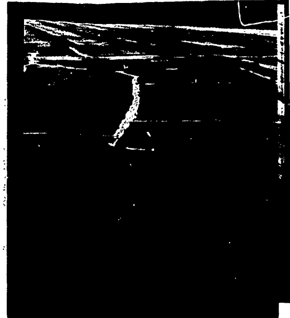
PHOTO 14 : SEALED TRANSVERSE AND LONGITUDINAL CRACKS ON
