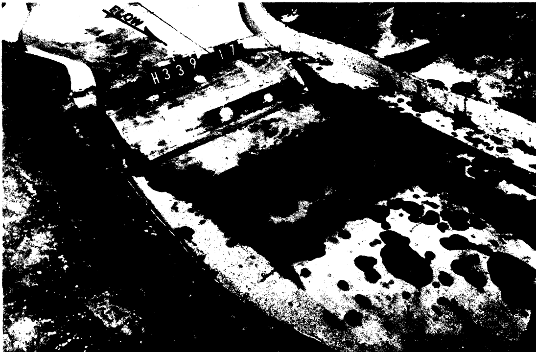
Photo 46. Drop 1, type 1 design stilling basin
