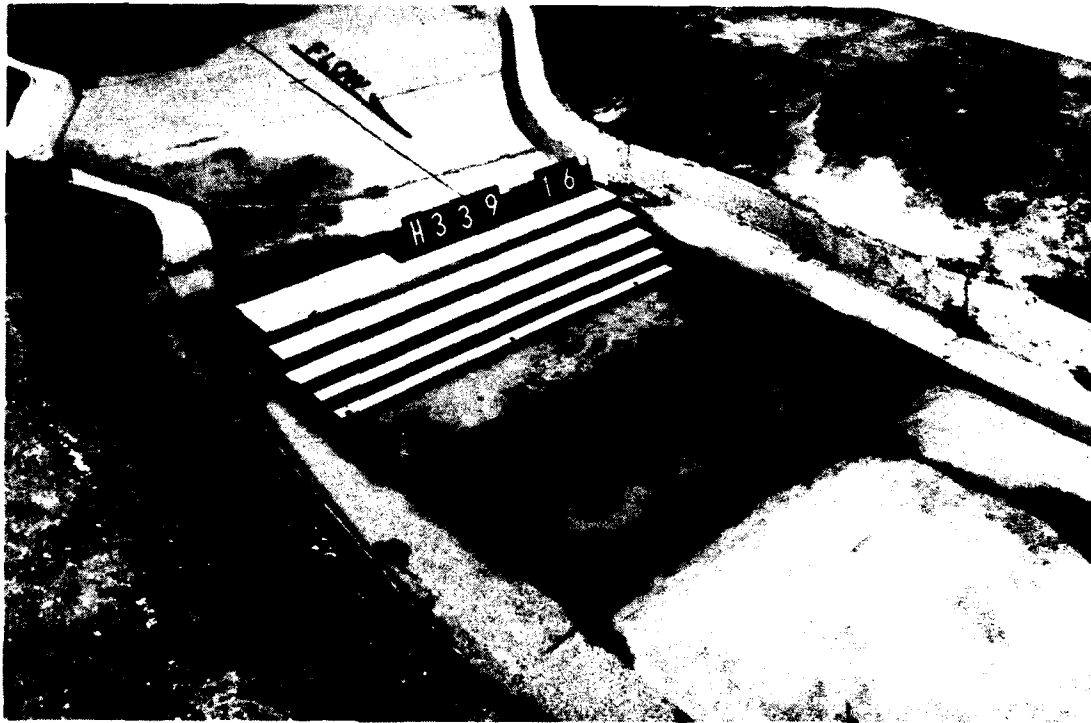
Photo 48. Drop 1, type 2 design stilling basin
