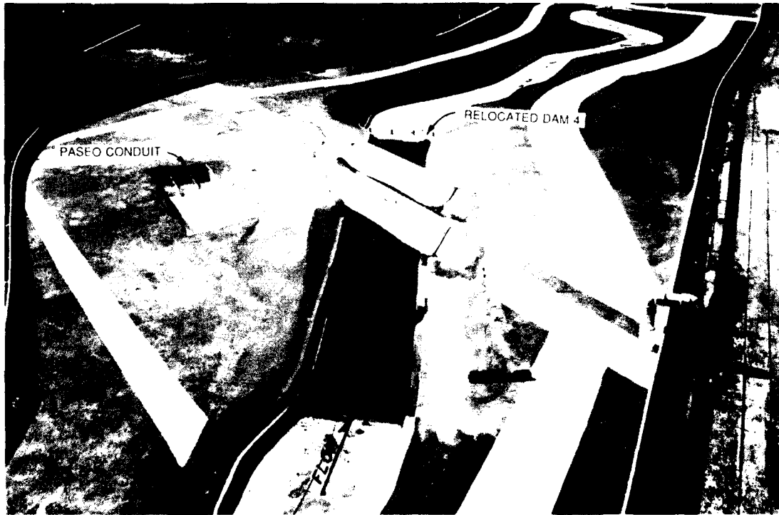
Photo 59. Paseo realignment, sta 123+00 to sta 147+00
