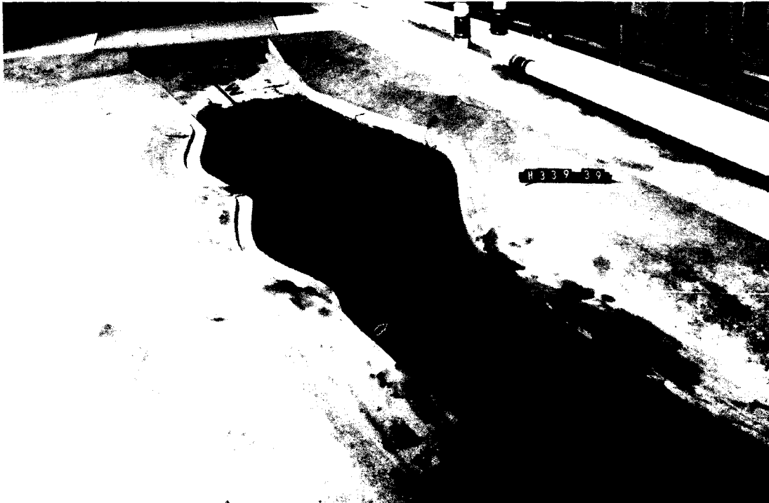
Photo 50. Drop 1, type 4 design stilling basin
