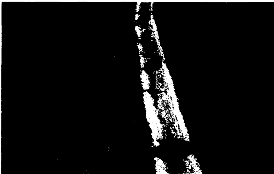
Figure 113. Thaw subsidence at ice wedges and cross drainage on road between well site and airfield at Itkillik.
