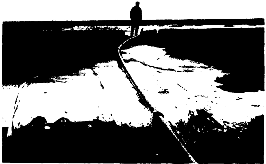
Figure 117. Washout of taxiway at Tunalik three years after construction. Fiberglass pipe placed during previous year to drain pond. Note membrane atop insulation.
