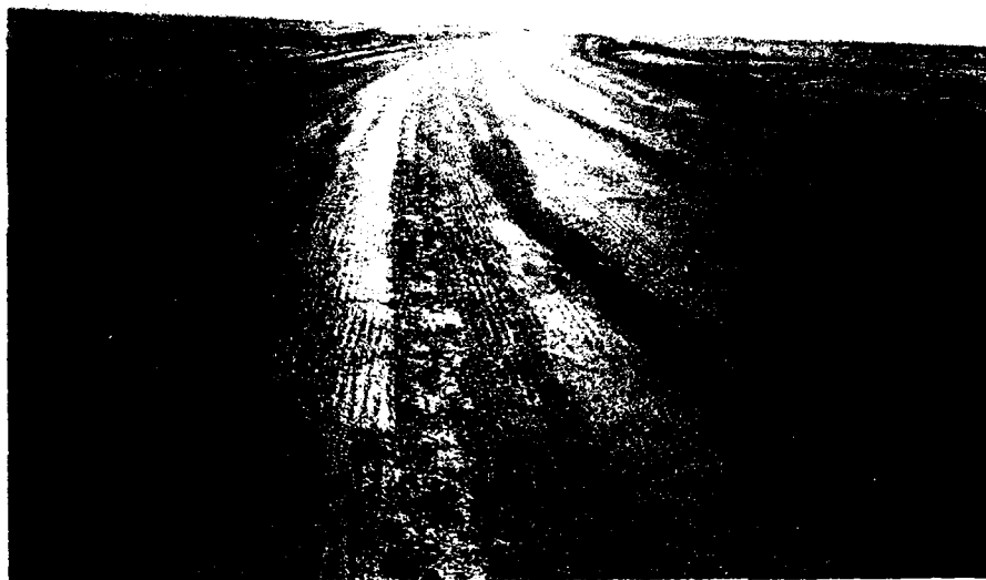
Figure 49. Ice road at Tunalik, scarified by grader for better traction.
