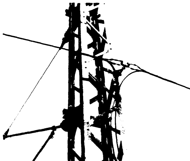
Fig. 5 Mid-span break-out with 2 dead-end spirals
