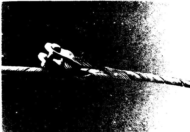
Fig. 6a Dead-end spiral for the F.O. aerial cable
