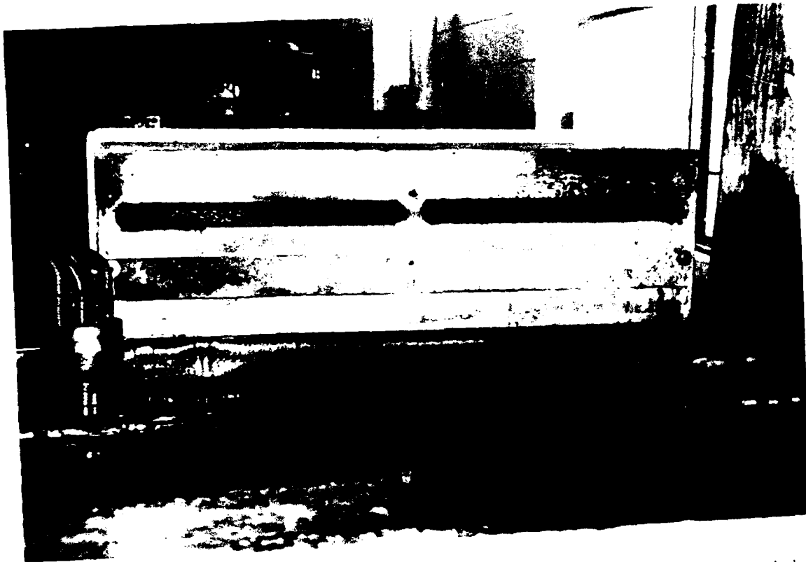
Figure B-9. Ventilation hood with one vent closed (tank lid was partially closed during operation).
