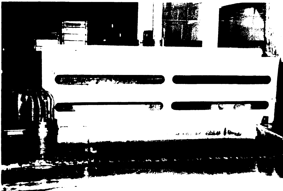
Figure B-8. Ventilation hood for chromic acid stripping tank (tank lid was partially closed during operation).
