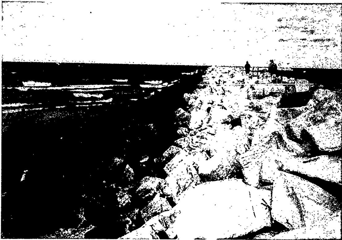
Figure 37. South breakwater, lakeside, 17 November 1988
