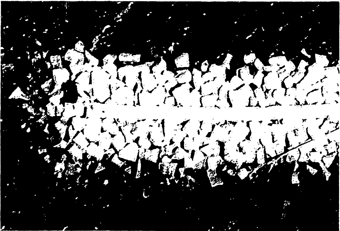
Figure 107. South breakwater head, 3 June 1986
